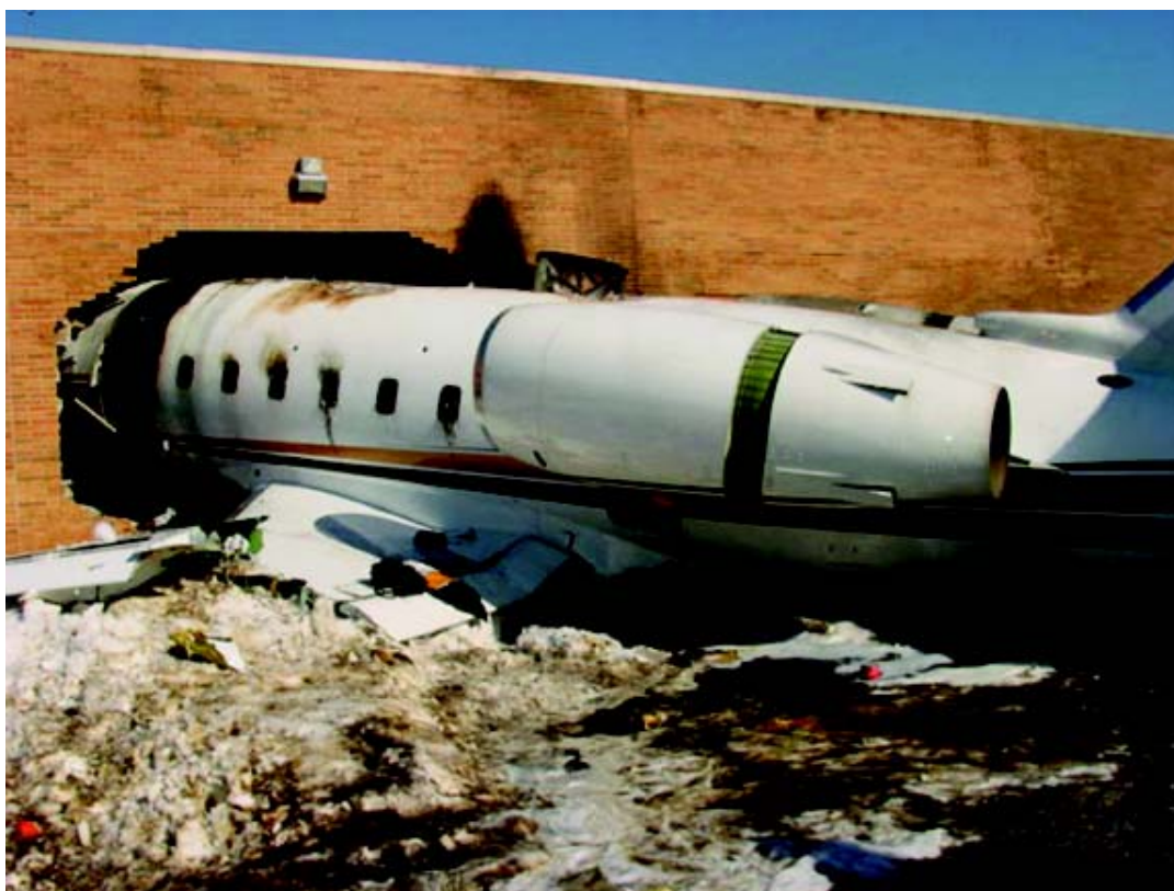
Figure 1. The airplane wreckage partially embedded in the building after the postimpact fire was extinguished.
