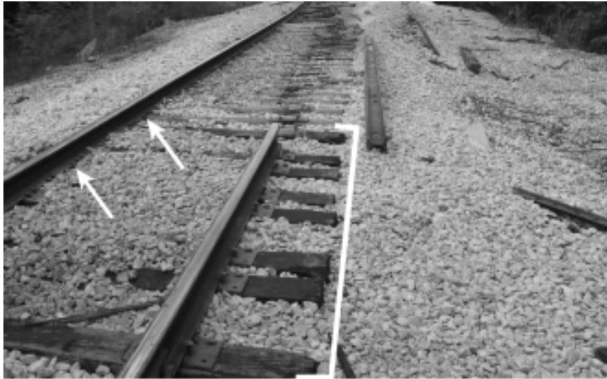
Figure 10. New ties with few anchors. Bracket indicates new ties. Arrows indicate anchors.
