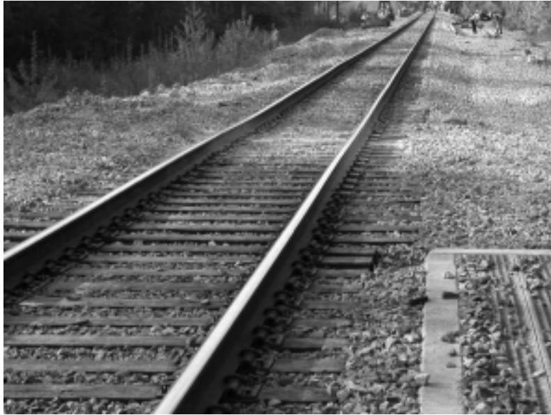
Figure 8. Fouled ballast.
