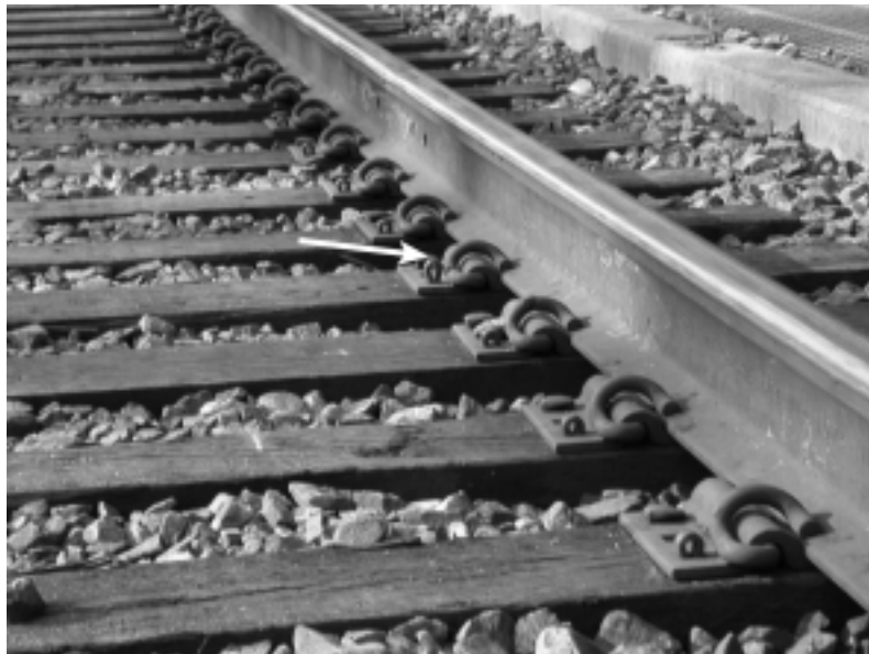
Figure 6. Elastic metal clip anchors.
