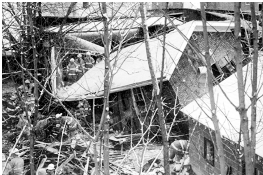
Figure 4. Destroyed residence where one fatal and one serious injury occurred.
