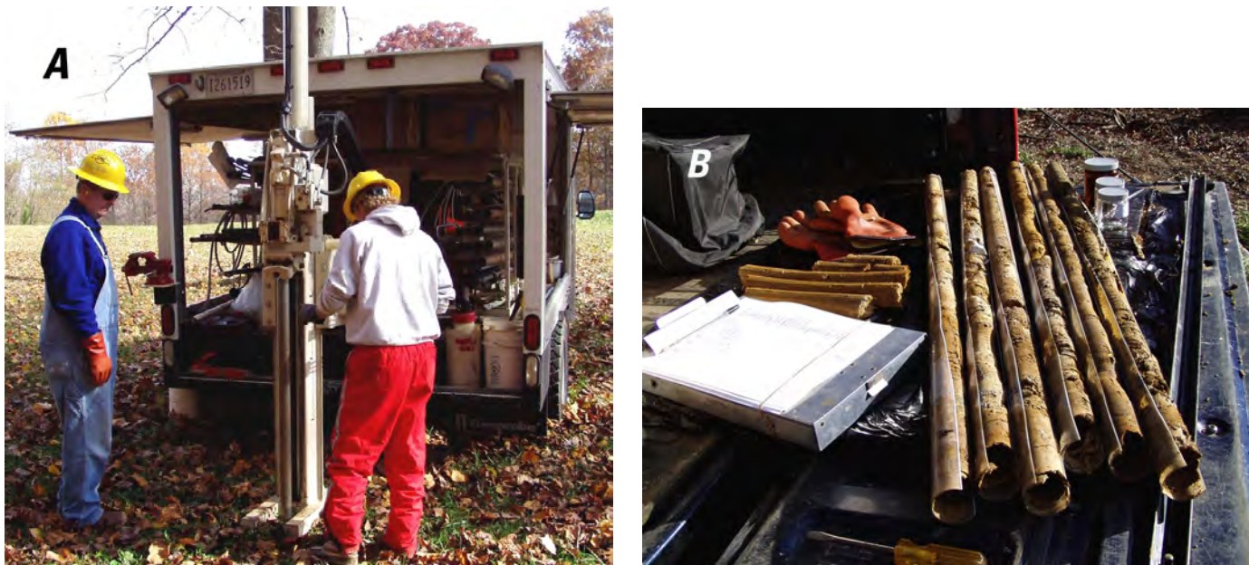
Figure 4. (A) Direct-push drill rig and (B) typical sediment cores collected at the Muscatatuck Urban Training Center near Butlerville, Indiana, October and November 2005.
