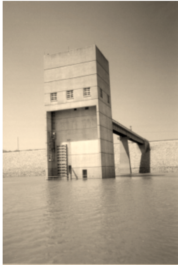
Figure 2. Salamonie Lake dam spillway tower.
