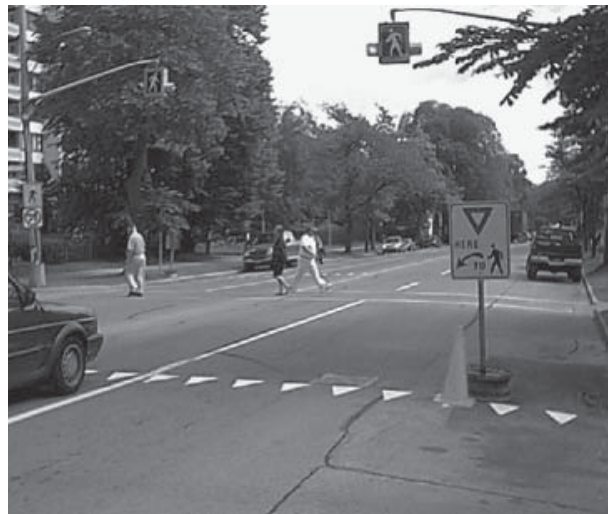
Advance yield markings
