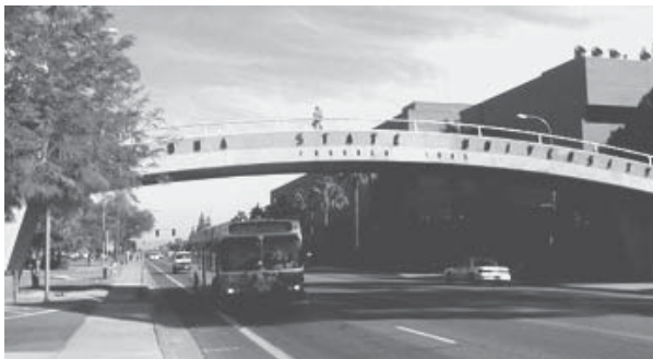
Existing pedestrian overpass in Tempe
