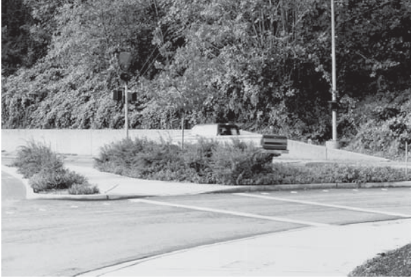
Right-turn slip lane with refuge island
