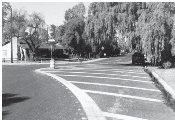
Narrowed street through the use of striping
