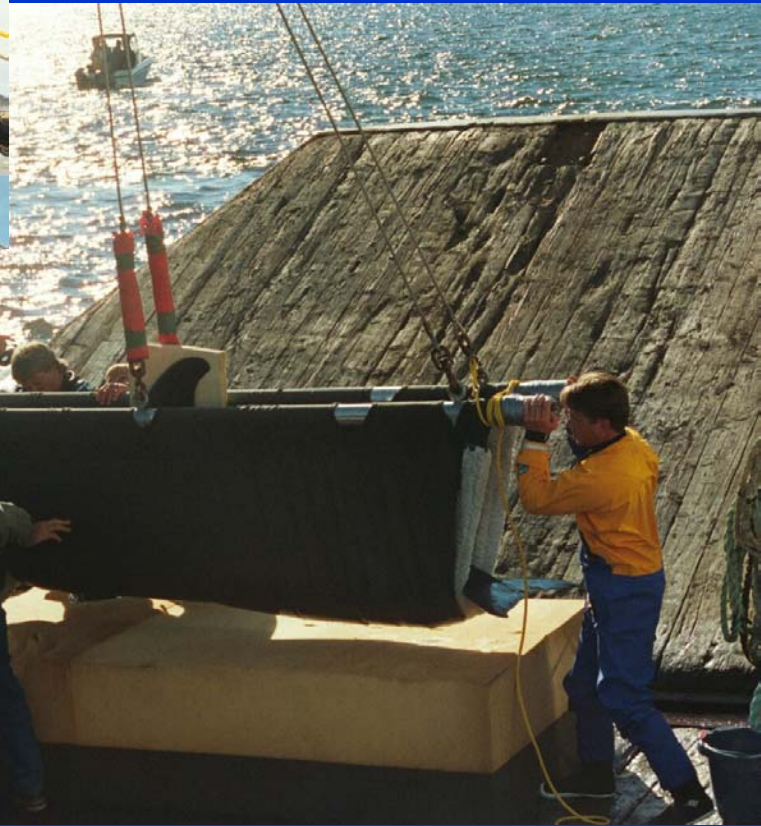
Lifted onto barge for short transport to new pen
