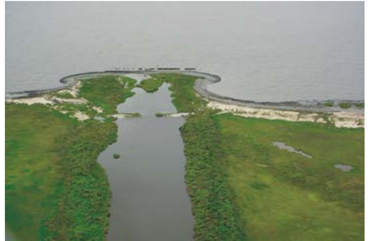
The beach where a pipeline canal meets the Gulf of Mexico has been stabilized with concrete mats thus preventing saltwater intrusion into the interior wetlands of Point au Fer Island.
