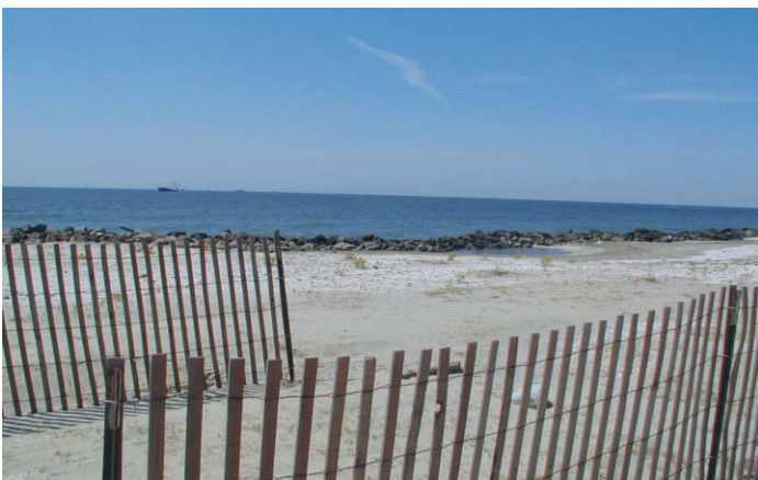
After dredged sediments were used to create dune and marsh habitats along East Timbalier Island, sand fences and vegetation were placed to stabilize the island's gulf shorelines.
