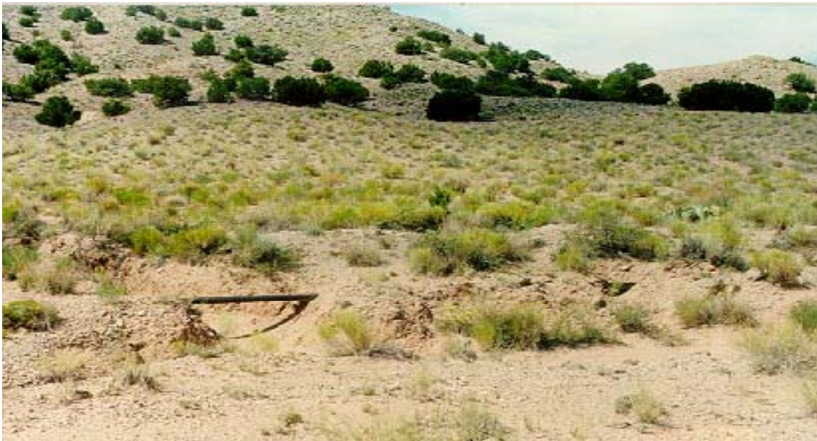
Photo 3. Erosion at abandoned pipeline
