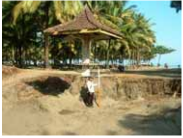
1.6m Scoured by Tsunami Turbulence
