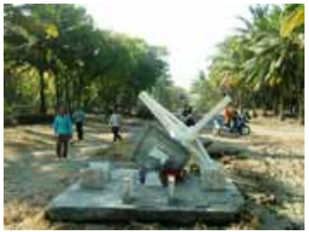
Shelter Toppled by Tsunami
