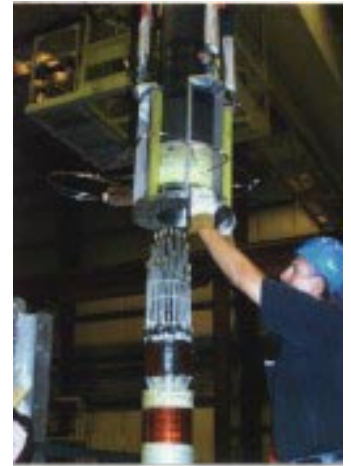
PPPL's Joe Bartzak assists as the OH coil is lowered over the center stack TF coil bundle.
