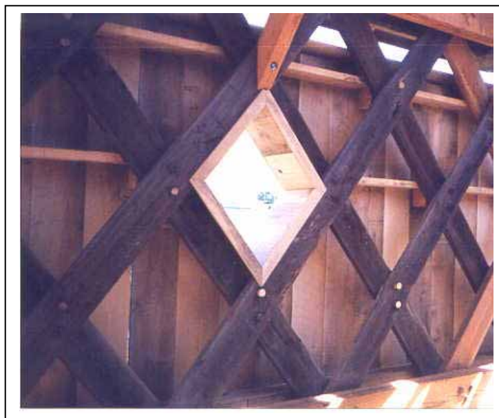
Figure 162. Good siding details around a window—Fitch's Bridge.
