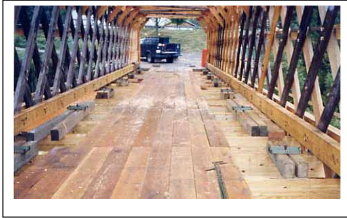
Figure 40. Transverse floor beams and longitudinal decking—Fitch's Bridge, Delaware County, NY.
