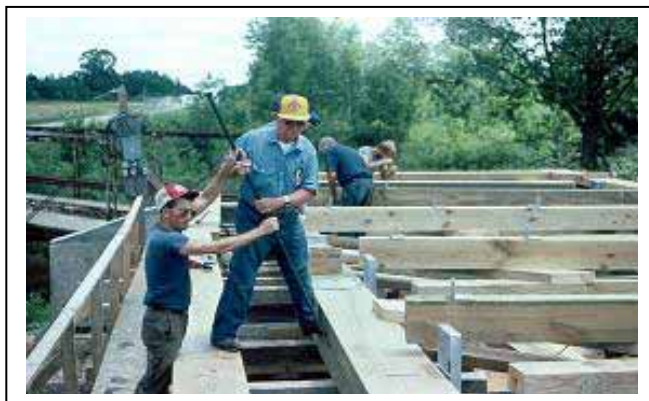
Figure 225. Truss assembly.
