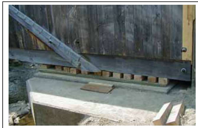
Figure 74. Bearing block installation—Brown's River Bridge, Westford, Vermont.
