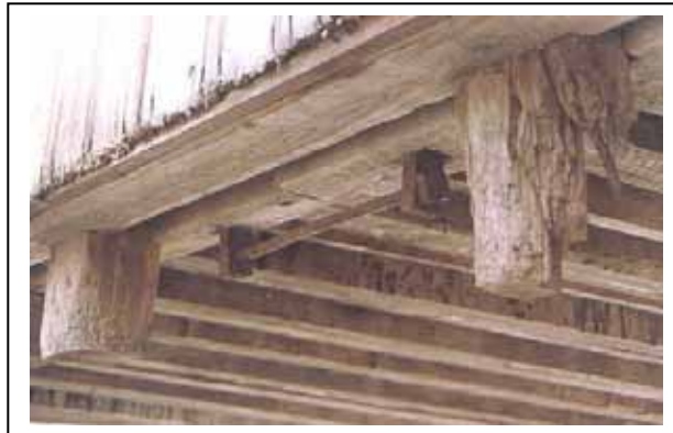
Figure 240. Bar-and-rod connector tensile splice.
