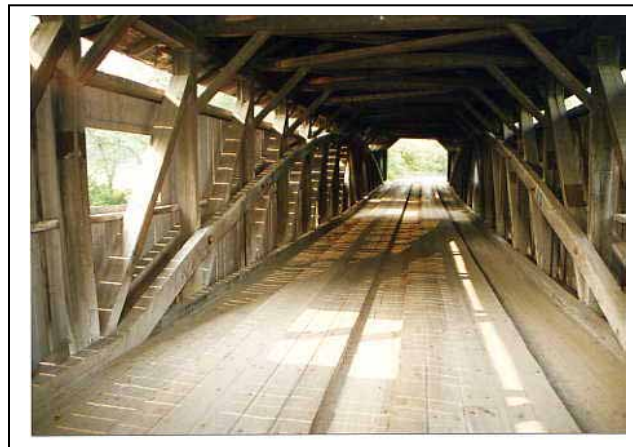
Figure 49. Running plank installation—Taftsville Bridge, VT.
