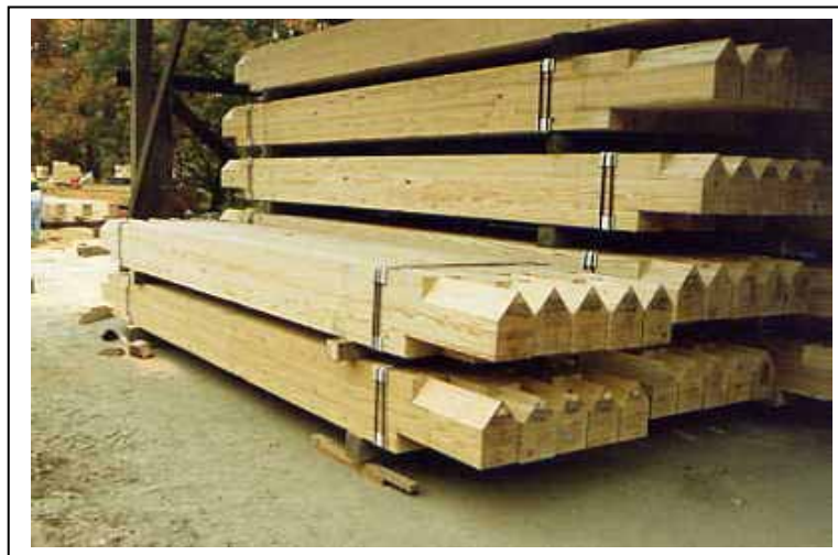
Figure 43. End notches of floor beams used in a Town lattice truss—West Dummerston Bridge, VT.
