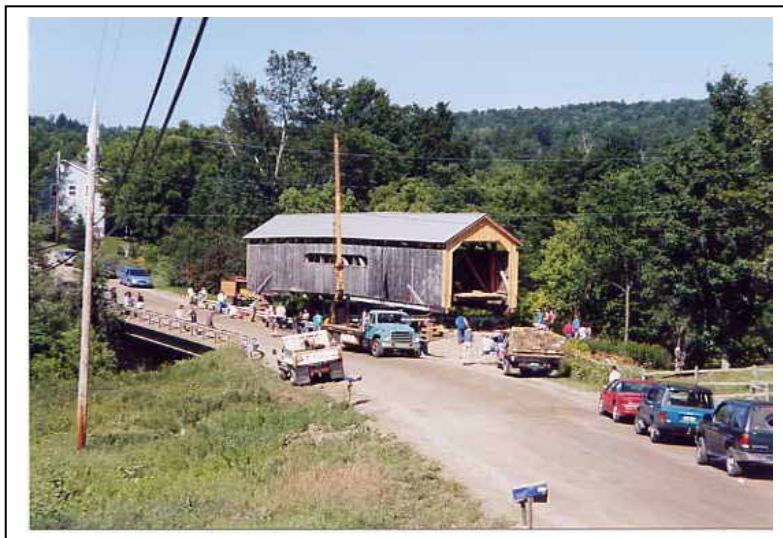
Figure 140. Brown's River Bridge, Westford, VT.
