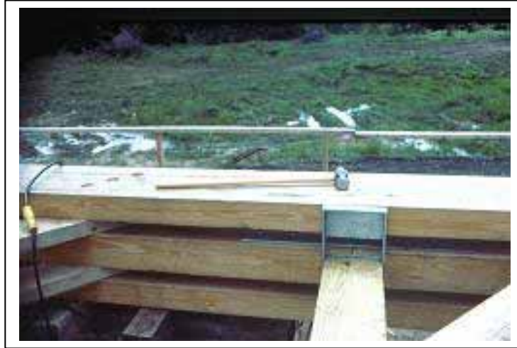
Figure 226. Three chord elements.
