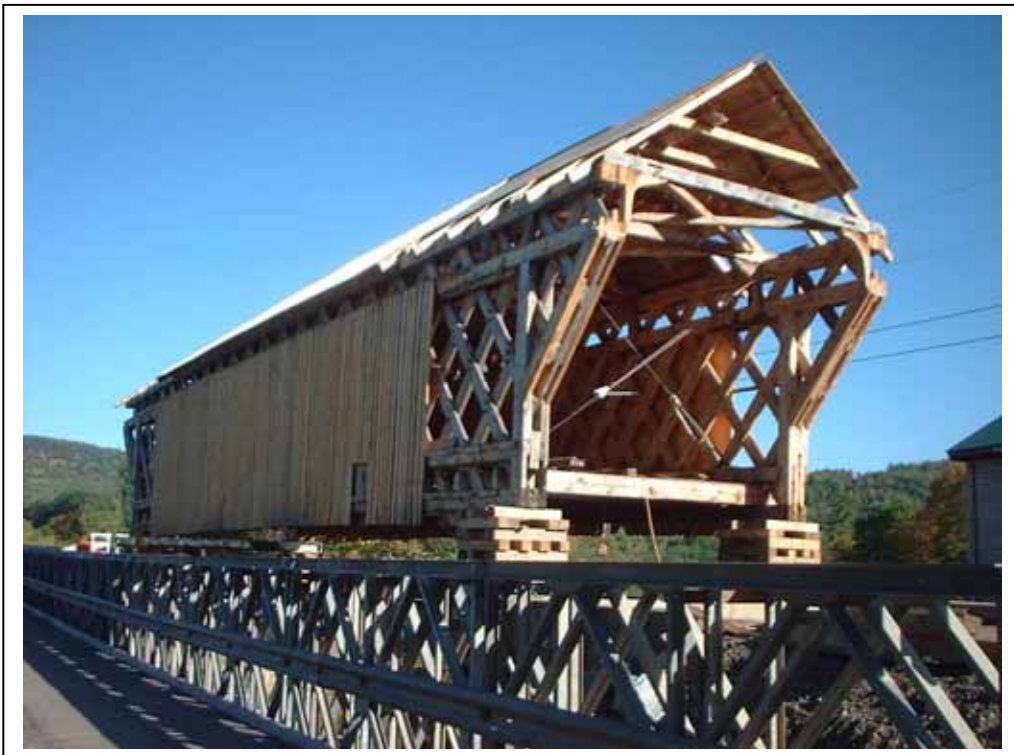
Figure 217. Bridge in place awaiting final lowering.
