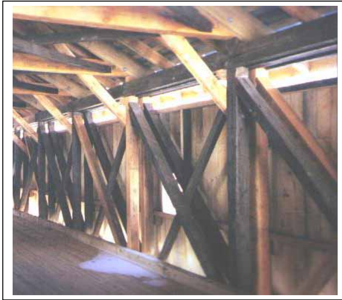
Figure 121. Long truss with counter timbers.
