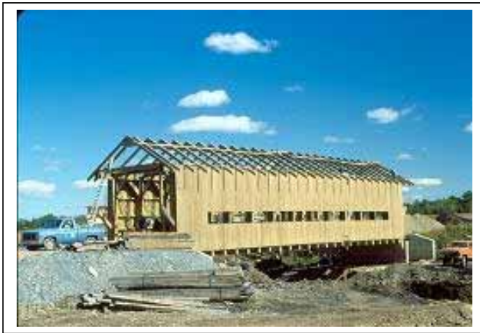
Figure 230. Installation of roof trusses and purlins.
