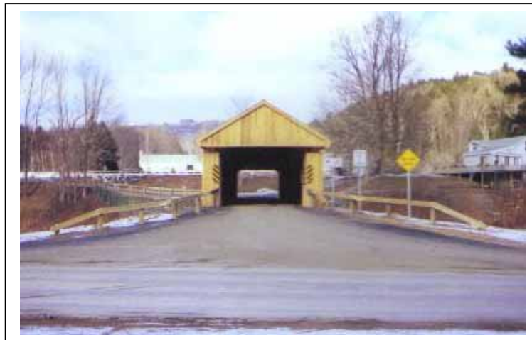
Figure 201. View of south entrance and railing configuration.
