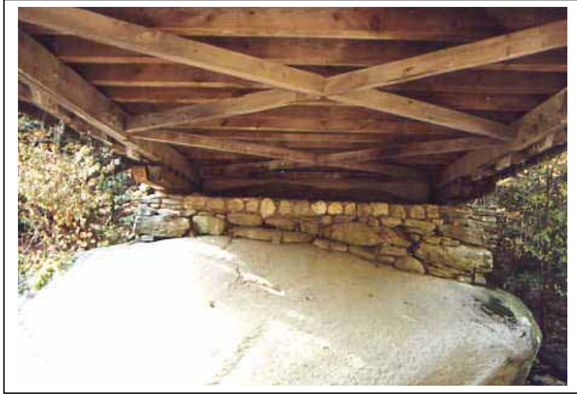
Figure 171. Brown Bridge, Shrewsbury, VT
