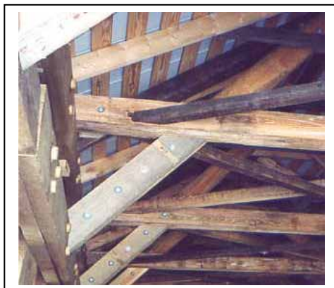
Figure 248. Modified knee braces.
