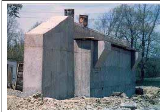
Figure 224. New stub abutment stem.
