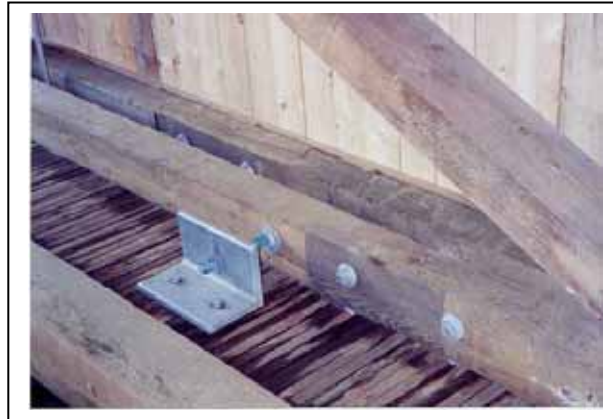
Figure 256. Connection between deck and bottom chord.
