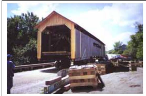
Figure 210. On top of the bypass bridge—ready to be slid sideways.
