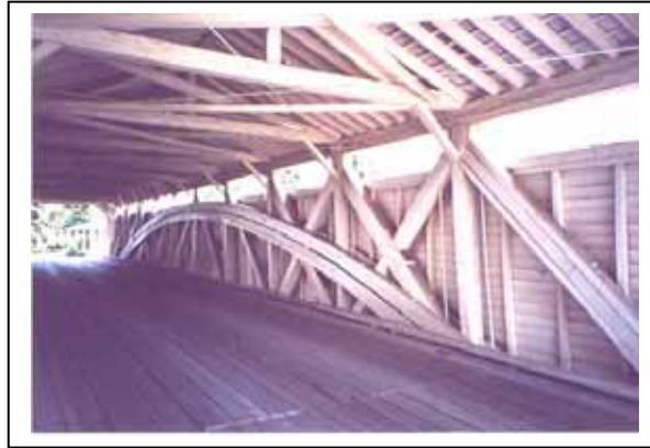
Figure 92. A heavy timber Burr arch–Wehr Bridge, Lehigh County, PA.
