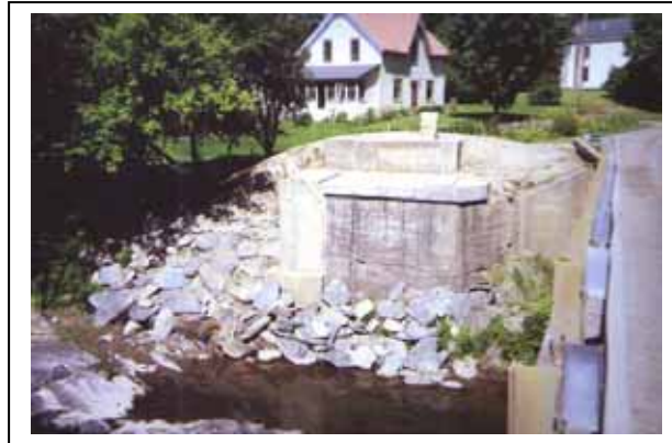
Figure 208. Reconstructed east abutment.
