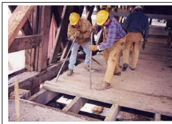
Figure 47. Nail-laminated decking being removed—Fitch’s Bridge, Delaware County, NY.
