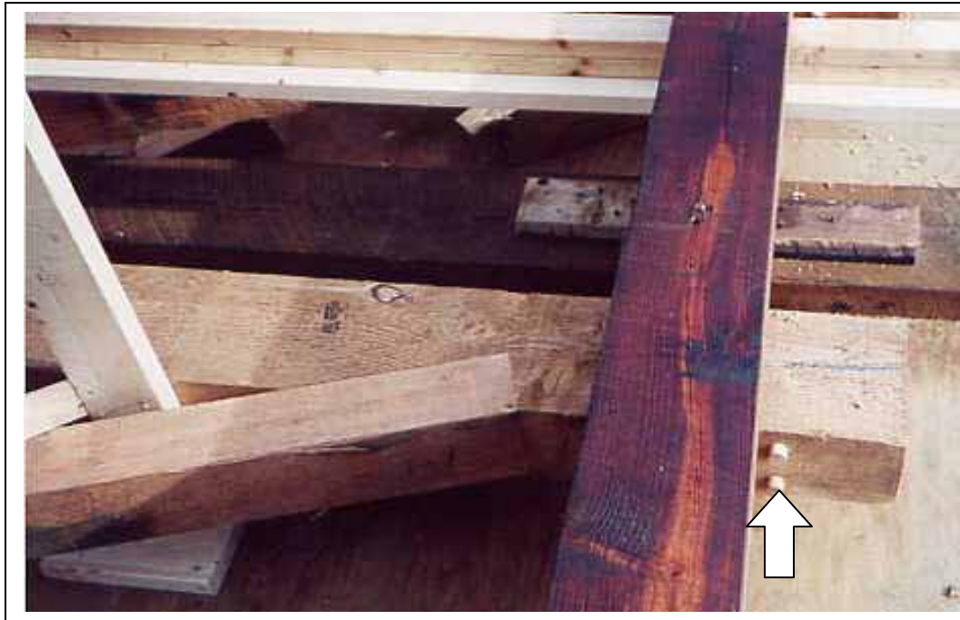
Figure 44. Timber dowel reinforcement of post-Mill Bridge, Tunbridge, VT.
