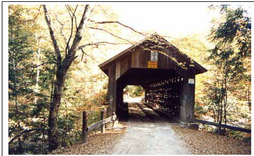
Figure 24. Brown Bridge—Shrewsbury, VT.
