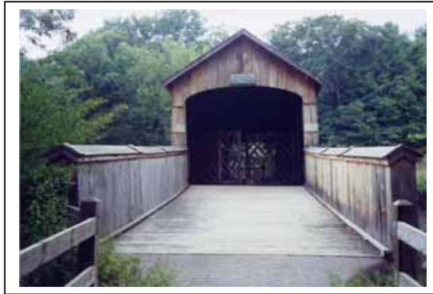
Figure 5. Pony truss covered bridge, Comstock Bridge, East Hampton, CT.
