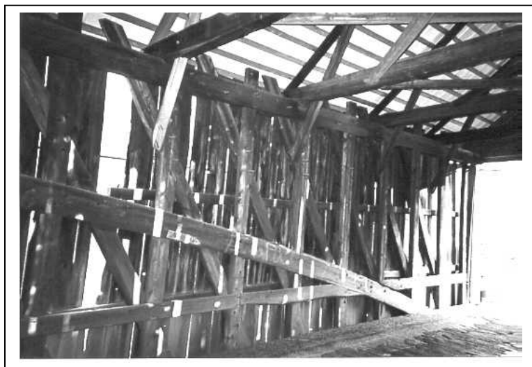
Figure 78. Thetford Center Bridge, interior view, Thetford, VT.
