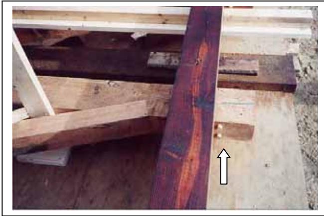
Figure 237. Wooden peg reinforcement of post corbel.
