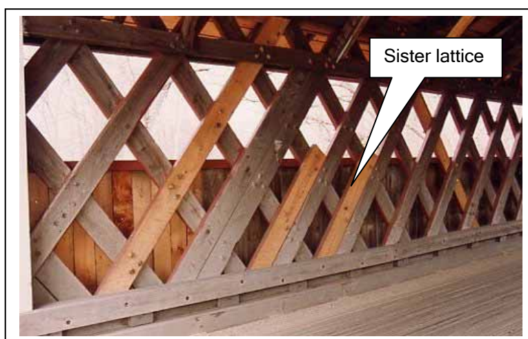
Figure 149. Sister elements in Town lattice—Silk Road Bridge, Bennington, VT.
