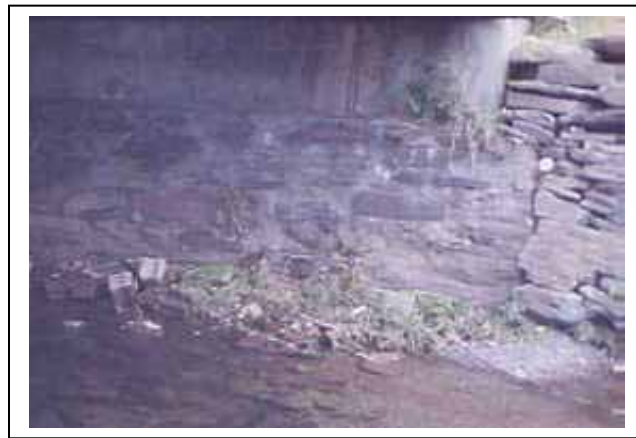
Figure 71. Parged stone abutment stem.
