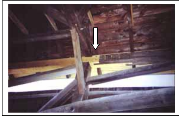
Figure 204. Replacement top chords.
