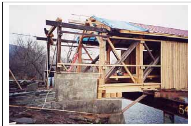
Figure 16. Framing of the independent shelter panel—Hamden Bridge, Delaware County, NY.
