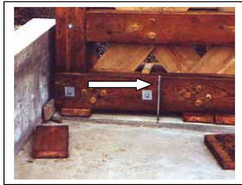
Figure 76. Hold-down anchor–Paper Mill Bridge, Bennington, VT.
