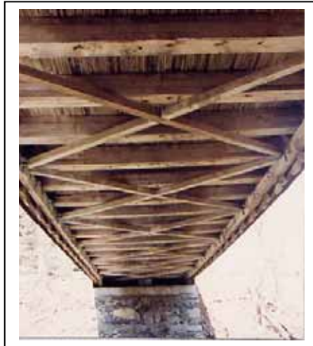
Figure 12. Lower lateral system—Williamsville, VT.
