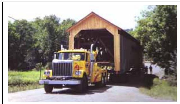
Figure 209. Underway on dollies.
