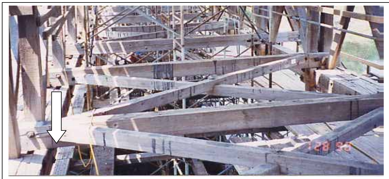
Figure 42. Mortise-and-tenon connection in floor beam—Downsville Bridge, Delaware County, NY.
