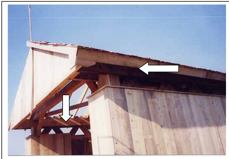
Figure 161. Good siding details—Fitch's Bridge, Delaware County, NY.
