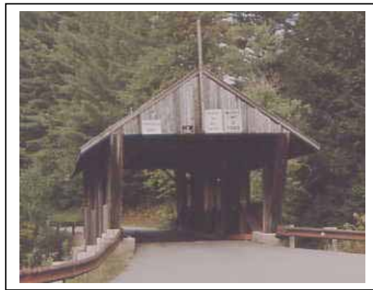
Figure 253. Bridge before collapse.
