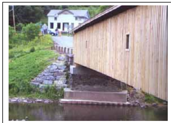
Figure 73. Modified original stone abutment—Fitch's Bridge, East Delhi, Delaware County, NY.
