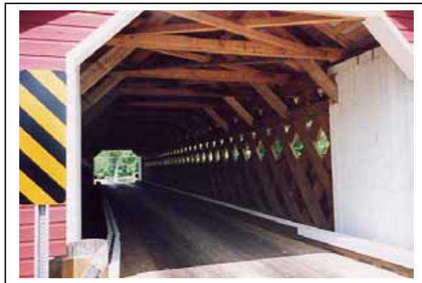
Figure 246. Entrance of completed bridge.
