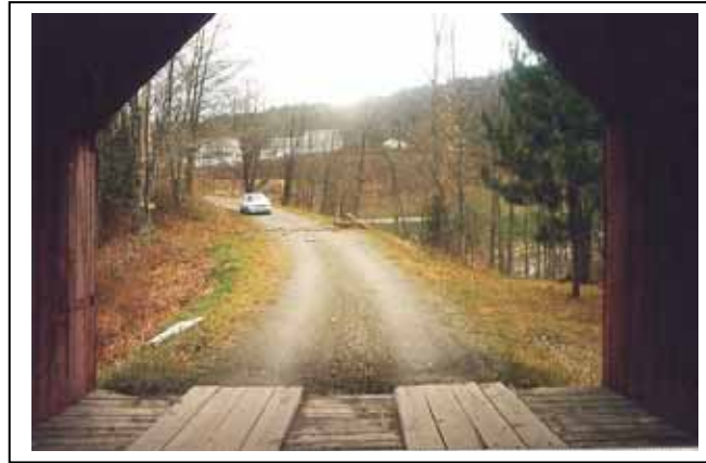
Figure 10. Running planks–Hutchins Bridge, VT.
