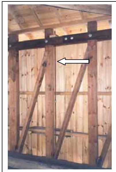
Figure 237. Wooden peg reinforcement of post corbel.
