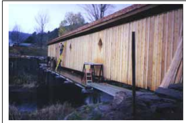
Figure 198. Siding details during installation.
