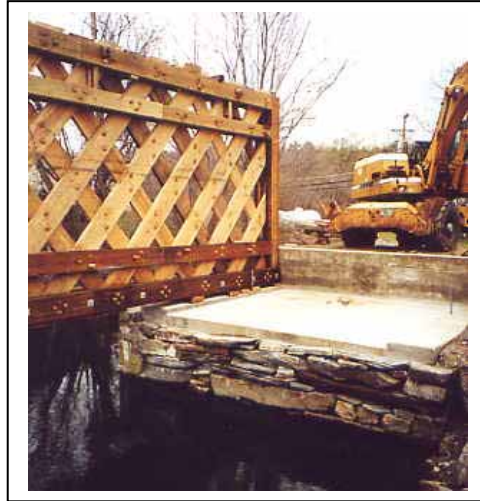
Figure 245. New pad at East Abutment—truss erection underway.
