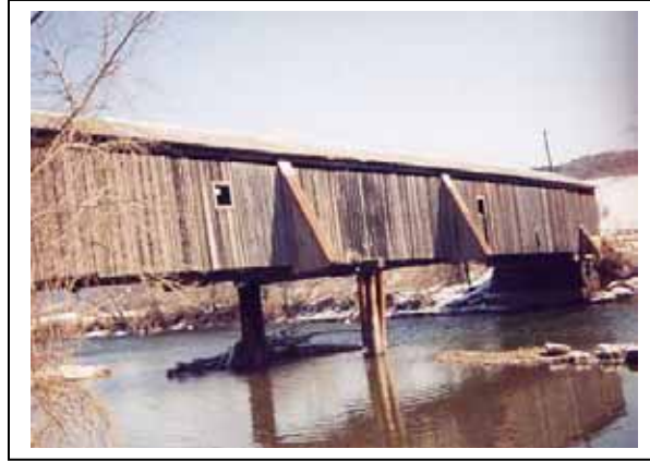
Figure 68. Supplemental pile bents—Hamden Bridge, Delaware County, NY.
