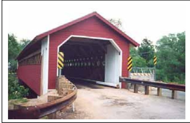
Figure 250. Bridge following reopening.
