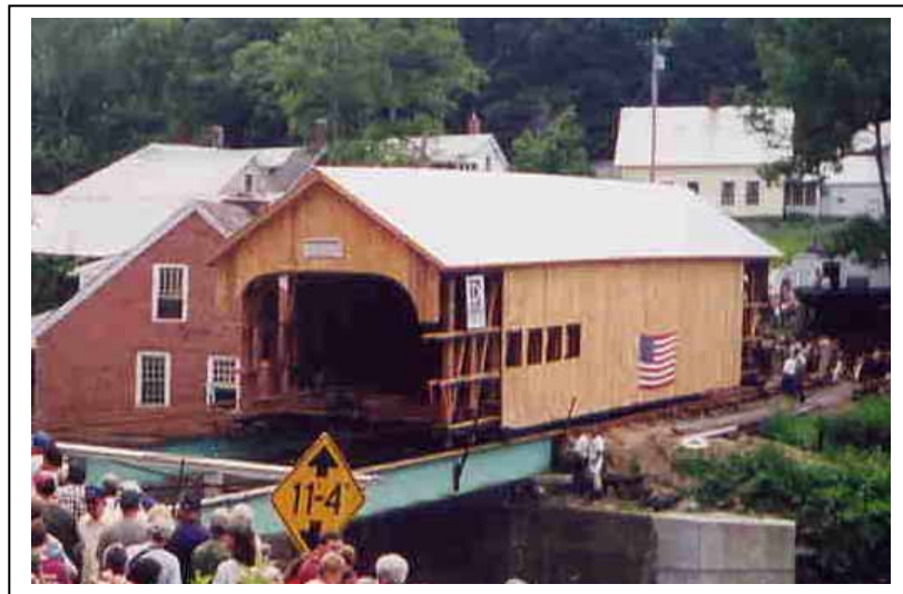
Figure 242. Bridge being moved into position.
