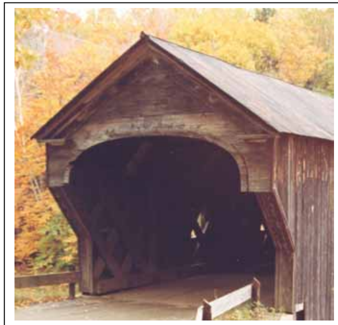
Figure 54. Unusual detailing of a portal—Upper Falls Bridge, Weathersfield, VT.
