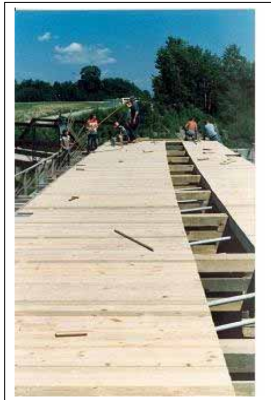
Figure 227. Adding siding before truss lifting and installation.
