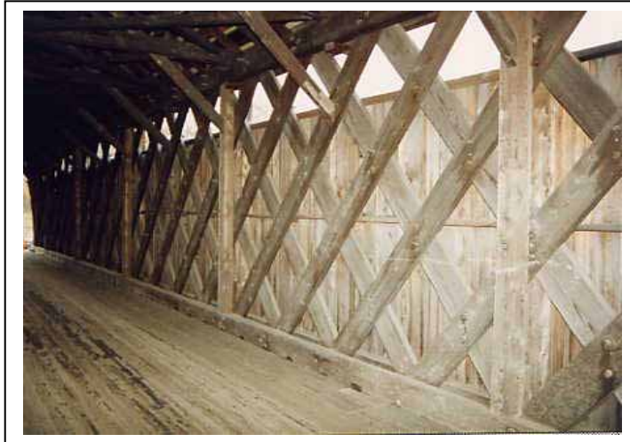
Figure 129. Intermediate posts—Worrall's Bridge, Rockingham, VT.
