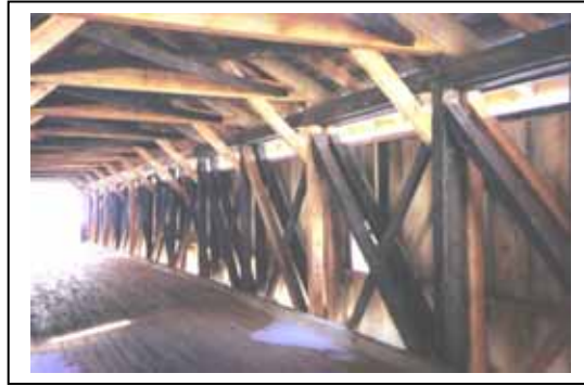
Figure 187. Final inside view. Note the lighter-colored replacement members.
