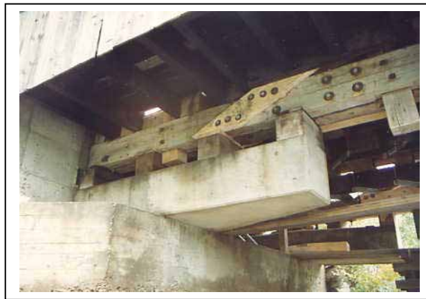
Figure 95. A bolster formed of concrete—Village or Great Eddy Bridge, Waitsfield, VT.
