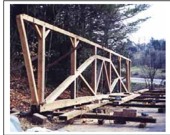
Figure 252. Completed replacement truss.
