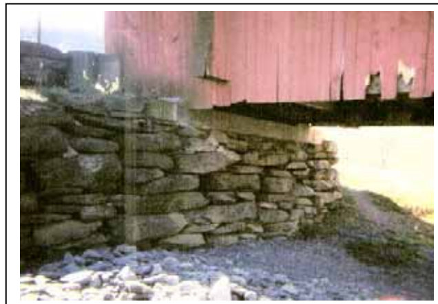
Figure 192. South Abutment prior to work.
