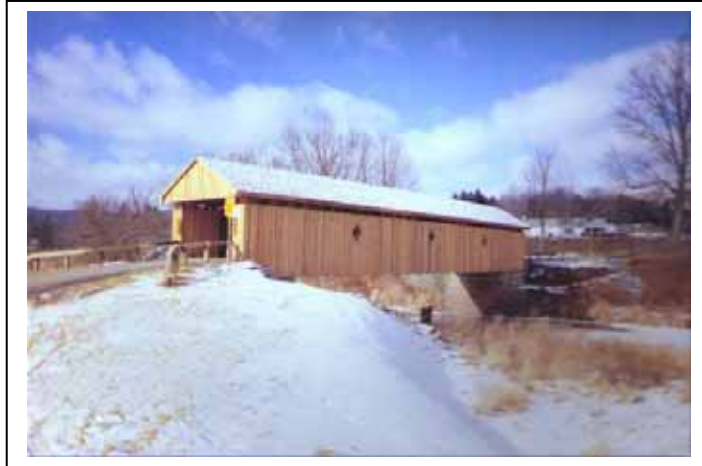
Figure 200. Elevation view of completed bridge.
