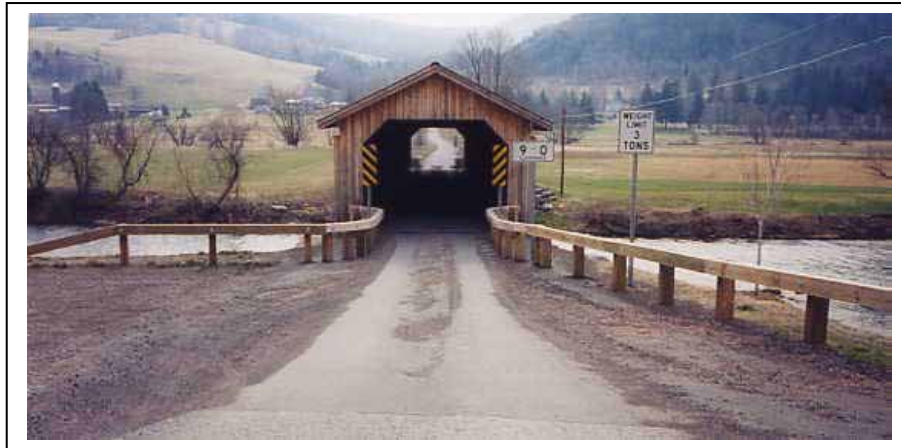
Figure 64. Squeeze timber approach railing—Hamden Bridge, Delaware County, NY.
