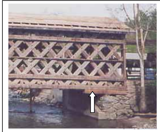
Figure 75. Bolster beam—Fuller Bridge, Montgomery, VT.
