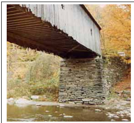
Figure 67. Original stone high abutment in good condition—Upper Falls Bridge, Weathersfield, VT.
