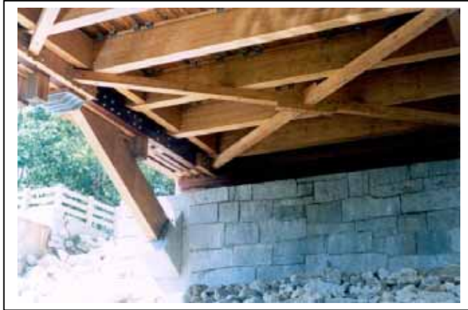
Figure 220. Underside of bridge showing floor beams, metal deck clips, bottom lateral bracing, arch springing area, and steel fabrication at the location where the arch passes through the bottom chord.
