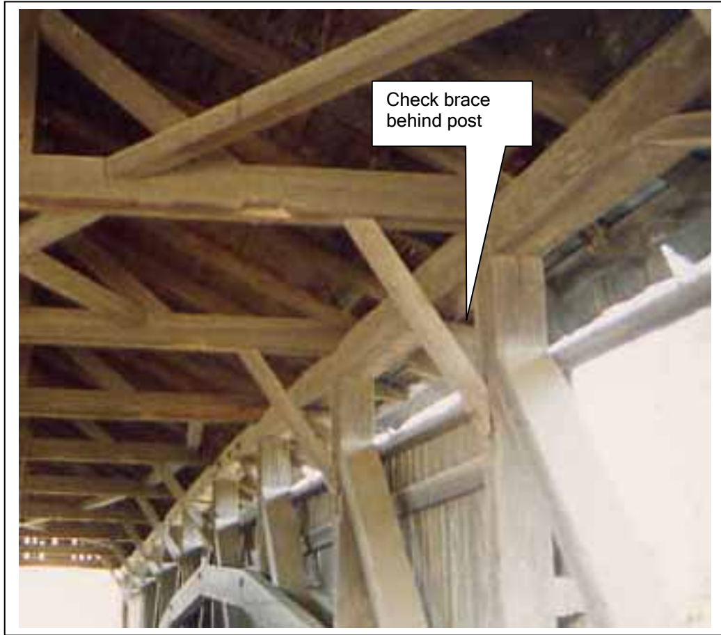
Figure 61. Check brace at top chord—Quinlan Bridge, Charlotte, VT.
