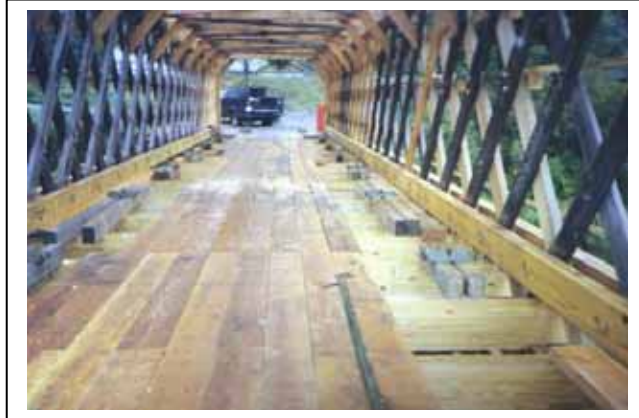
Figure 196. Partially installed deck.
