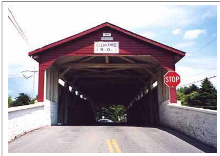
Figure 55. Example of portal extension–Wehr Bridge, Lehigh County, PA.
