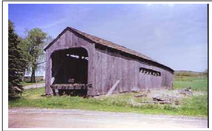
Figure 203. As the bridge sat for 13 years.
