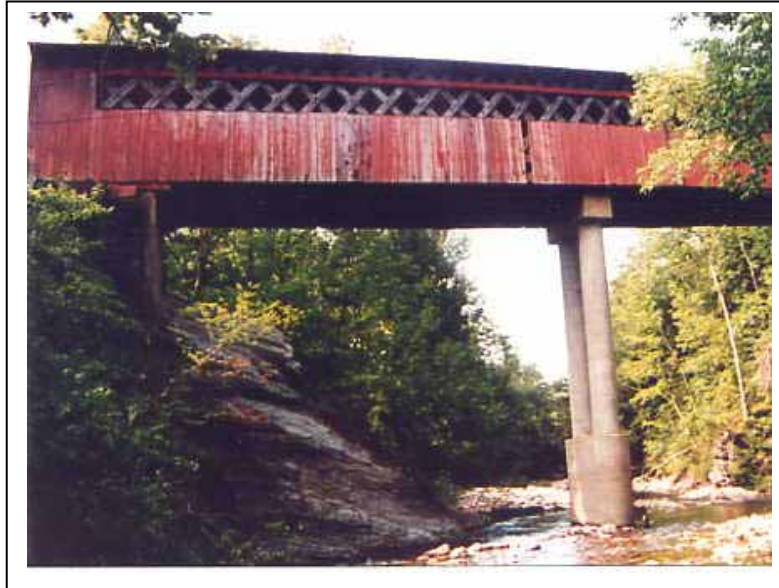
Figure 1. Chiselville Bridge, Sunderland, VT.
