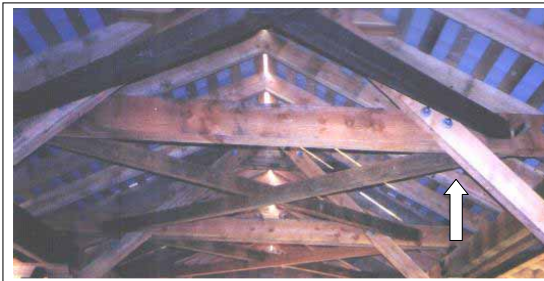
Figure 58. Alternative and stronger style of knee brace—Hamden Bridge, Delaware County, NY.
