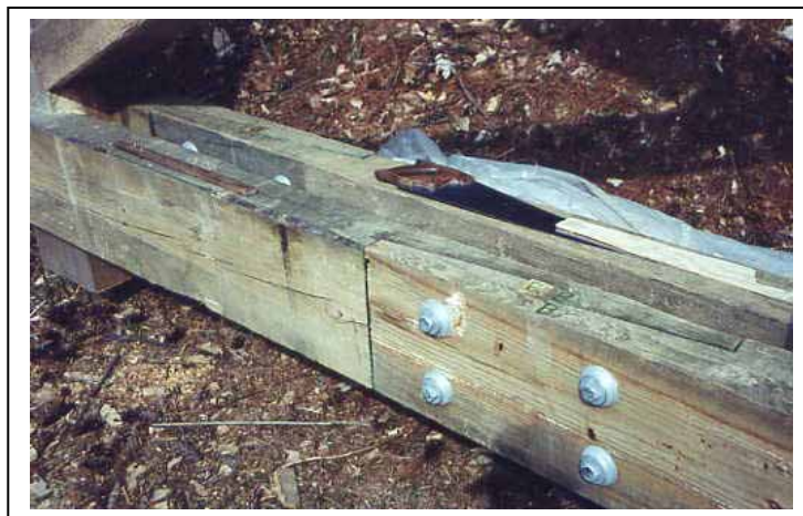
Figure 255. Double bottom chord arrangement with scarf joint.
