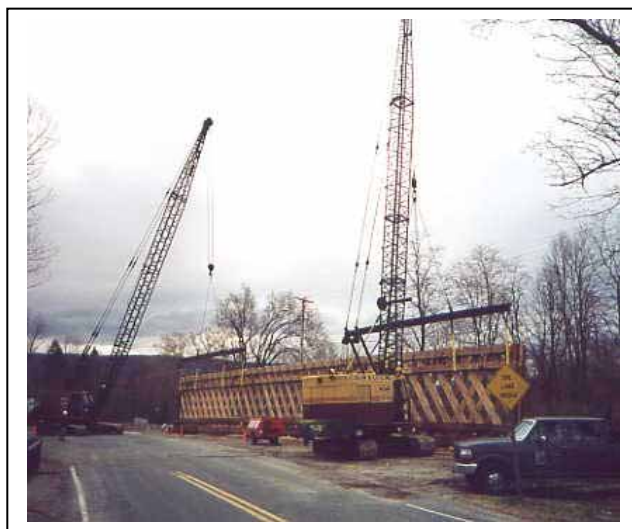
Figure 249. Cranes and truck positioning the trusses.
