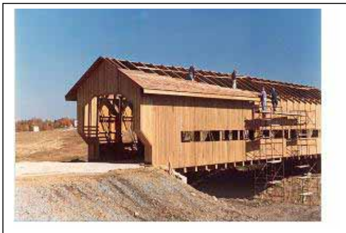
Figure 231. Installation of wood shingles.
