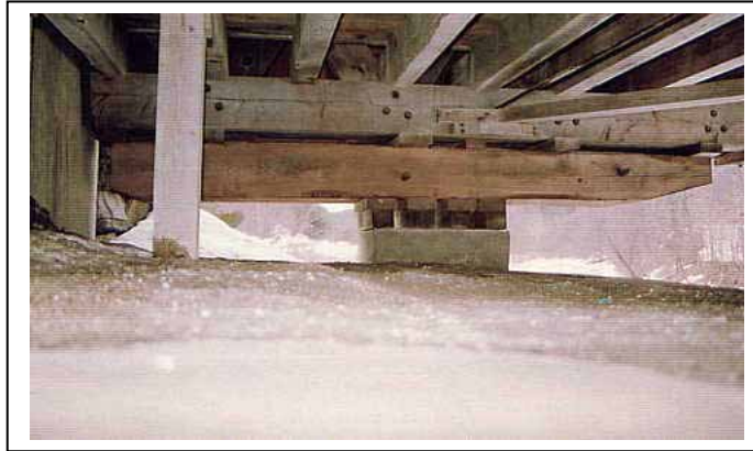
Figure 94. Large bolster beam supported on bearing blocks—Hall Bridge, Rockingham, VT.
