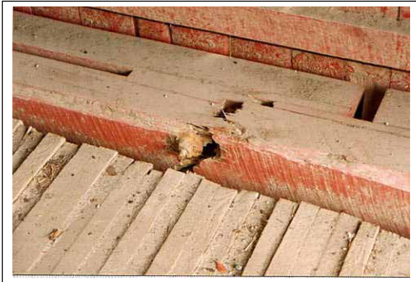
Figure 172. Lower Cox Bridge, Northfield, VT
