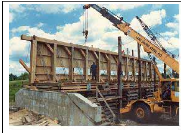
Figure 228. North truss in position and secured.
