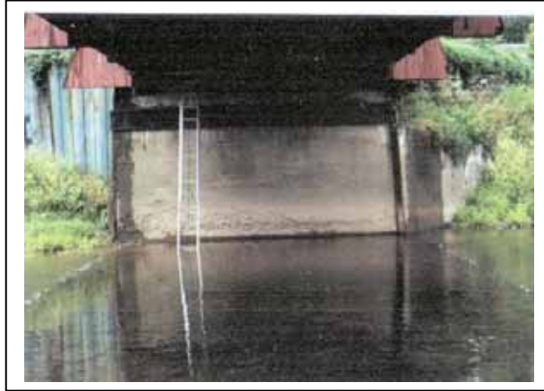
Figure 193. North Abutment prior to work.
