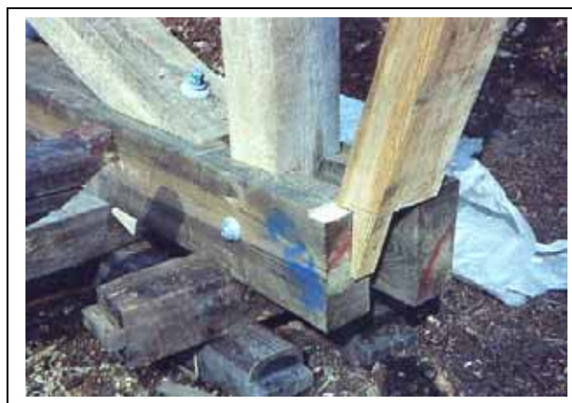
Figure 257. Heel connection details.
