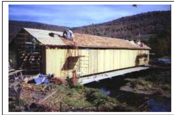
Figure 197. Installing cedar shakes.
