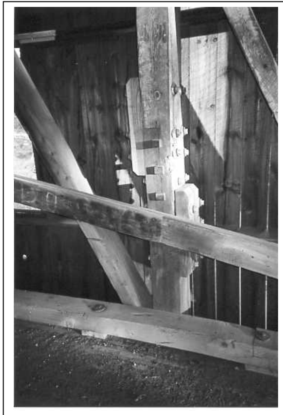
Figure 151. Partial post replacement in multiple kingpost truss—Union Village Bridge, VT.
