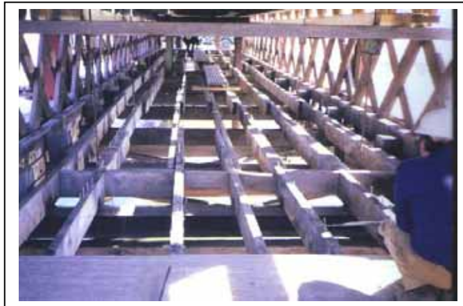
Figure 191. Partially removed 1976 floor.
