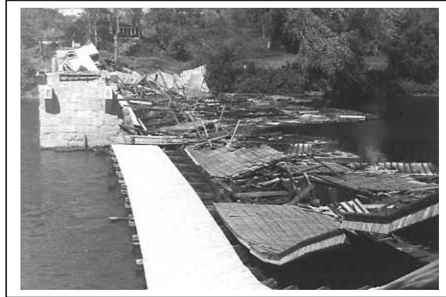
Figure 86. A covered bridge destroyed by wind—Bedell Bridge between Haverhill, NH, and Newbury, VT, 1979.
