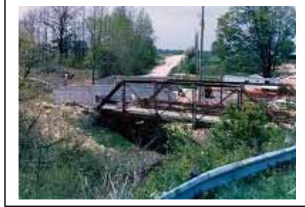
Figure 223. New abutment construction on new alignment.
