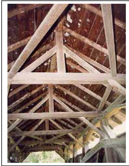
Figure 11. An unusual upper lateral system—Seguin Bridge, VT.
