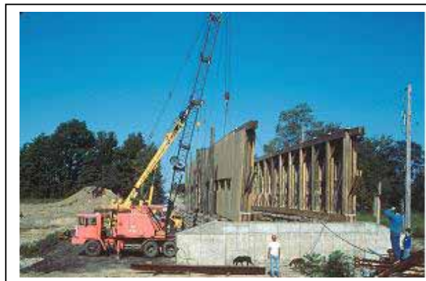
Figure 229. Both trusses erected.
