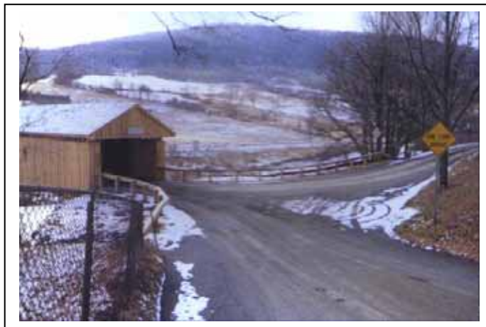
Figure 199. Approach railing configuration at north entrance.
