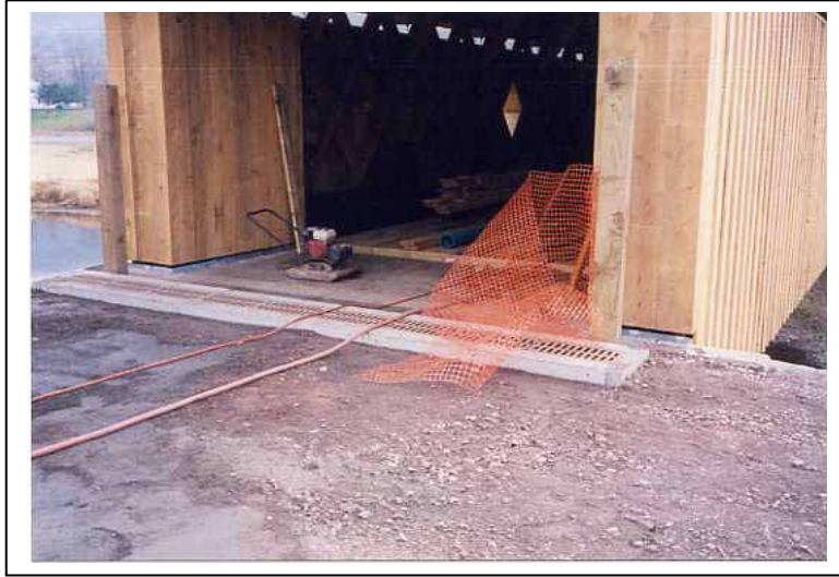
Figure 165. A trench drain at a bridge entrance—Fitch's Bridge, Delaware County, NY.
