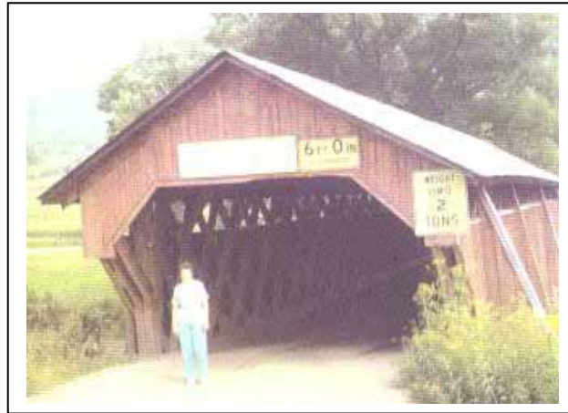
Figure 190. Older “hung” floor.
