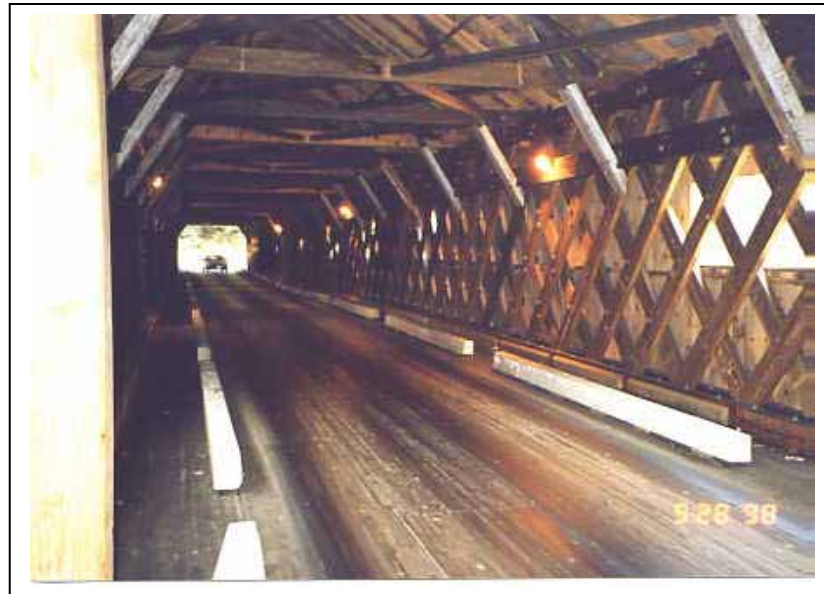
Figure 63. Interior curbing—West Dummerston Bridge, VT.
