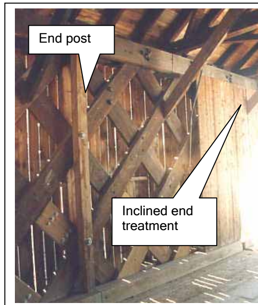
Figure 128. The corresponding interior end post—Bartonsville Bridge, Rockingham, VT.
