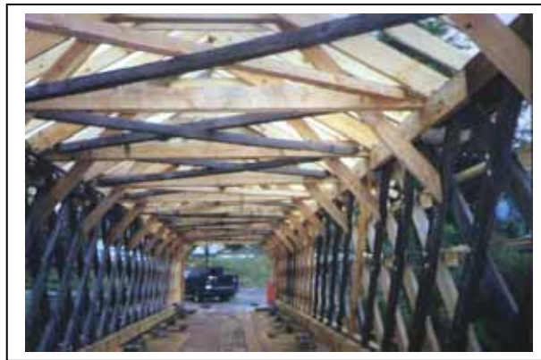
Figure 195. Reworked internal bracing system.
