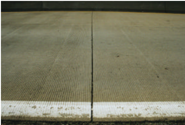
Figure 3.1.25 Close-up of distress free transverse joint at 39-3801.
