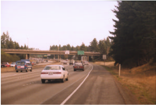
Figure 3.1.30 Overview of test site 53-3812.
