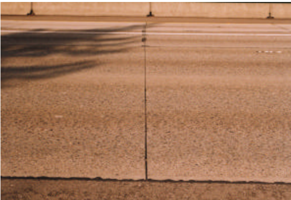
Figure 3.1.31 Close-up of a distress free transverse joint at 53-3812.
