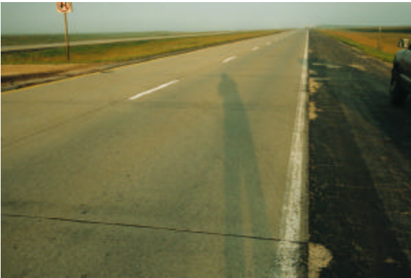
Figure 3.1.20 Typical distress free slab at 19-3055.
