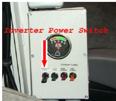
Figure 2.2.5.6. Remote switch for inverter power.
