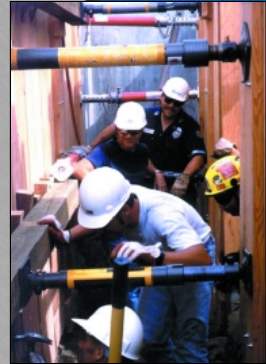
Workers in a 40-hour trench rescue class learn proper shoring and stabilization techniques as they attempt to rescue individuals trapped by a simulated cave-in.
