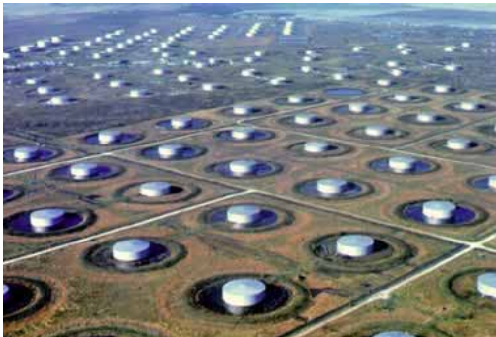
Figure 10.—An oil tank farm associated with the oil refining industry. The area is in League-Urban land complex, 0 to 1 percent slopes.
