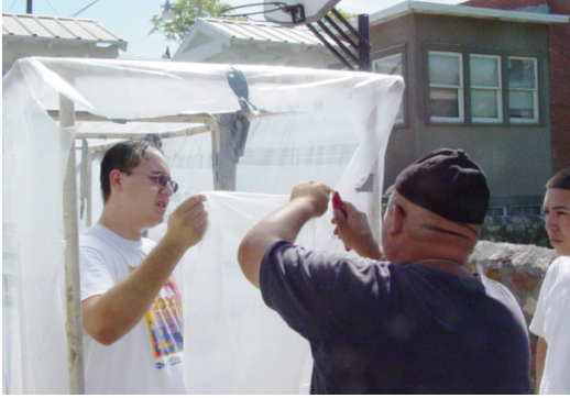
Building containment during asbestos training, HMTRI, El Paso, TX
