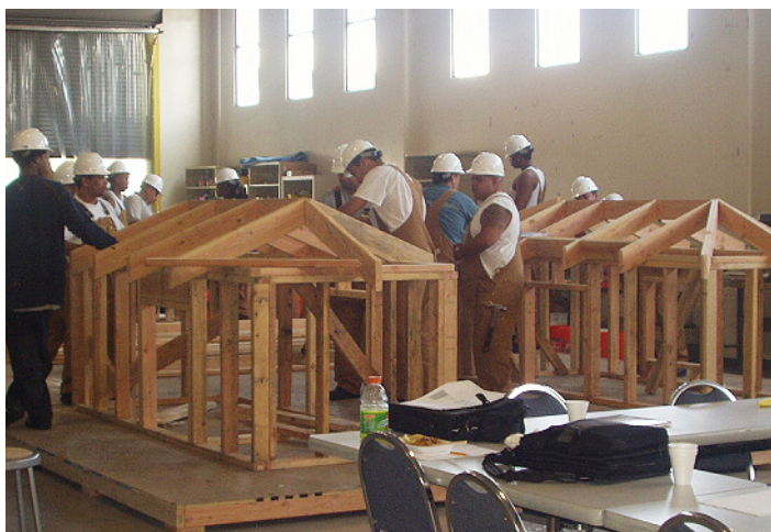
East Palo Alto BMWTP Program students built mockups of a home. Modules are assembled into a miniature house.
