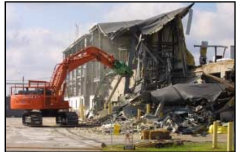
Demolition work at Savannah River.
