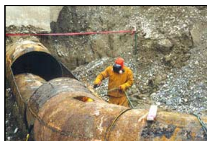
Hanford worker cutting a contaminated pipe.
