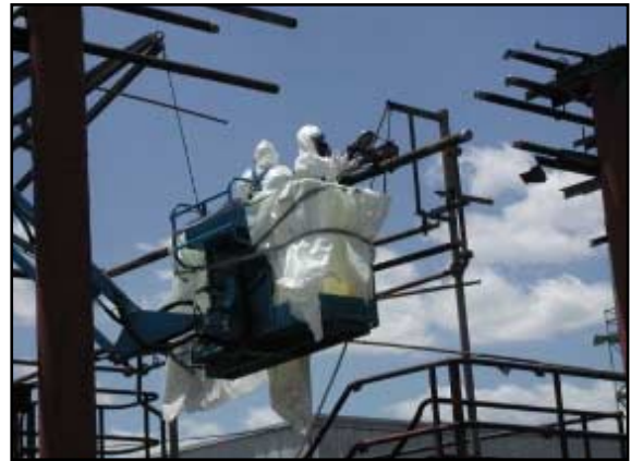
Cutting overhead pipe at Paducah
