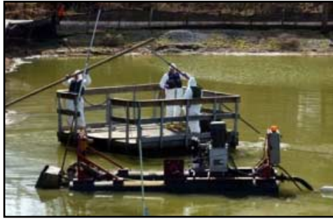
Dredging contaminated sediments at Oakridge National Laboratories
