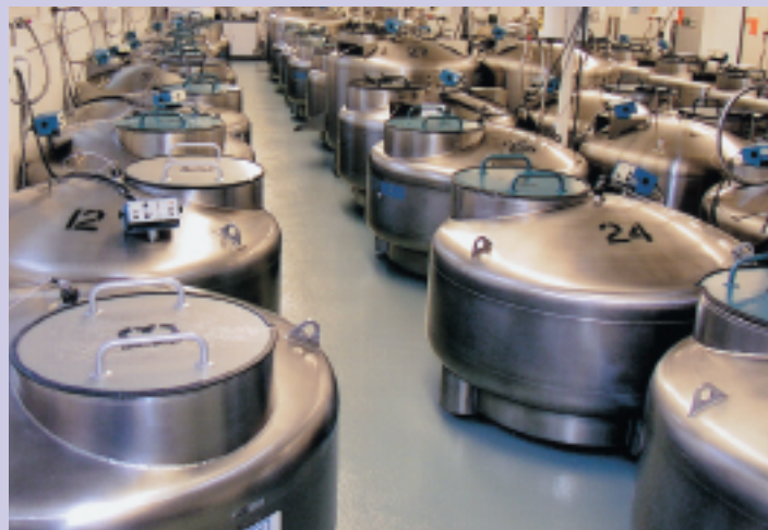
Main liquid nitrogen storage facility at Coriell
