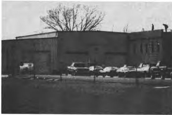
CrownLine Boats, Inc. is located in West Frankfort, IL. The company received an initial $104,000 RLF loan and two additional loans for working capital ($46,000 and $73,000). These three loans combined leveraged $2.87 million of private funding, $1.2 million of other public funding, and $31,200 of new equity. At the time of the first loan (1993), the company employed 200 people. Currently this number has increased and reaches 540.
