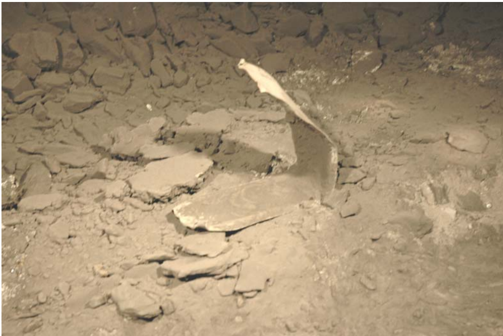
Photograph 8 - Middle segment of roof strap found in No. 5 Entry
