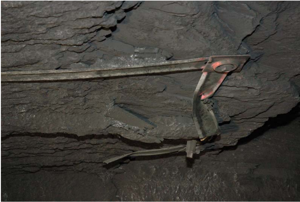
Figure 2 - Roof Straps at the No. 3 Seal Location for A Left
