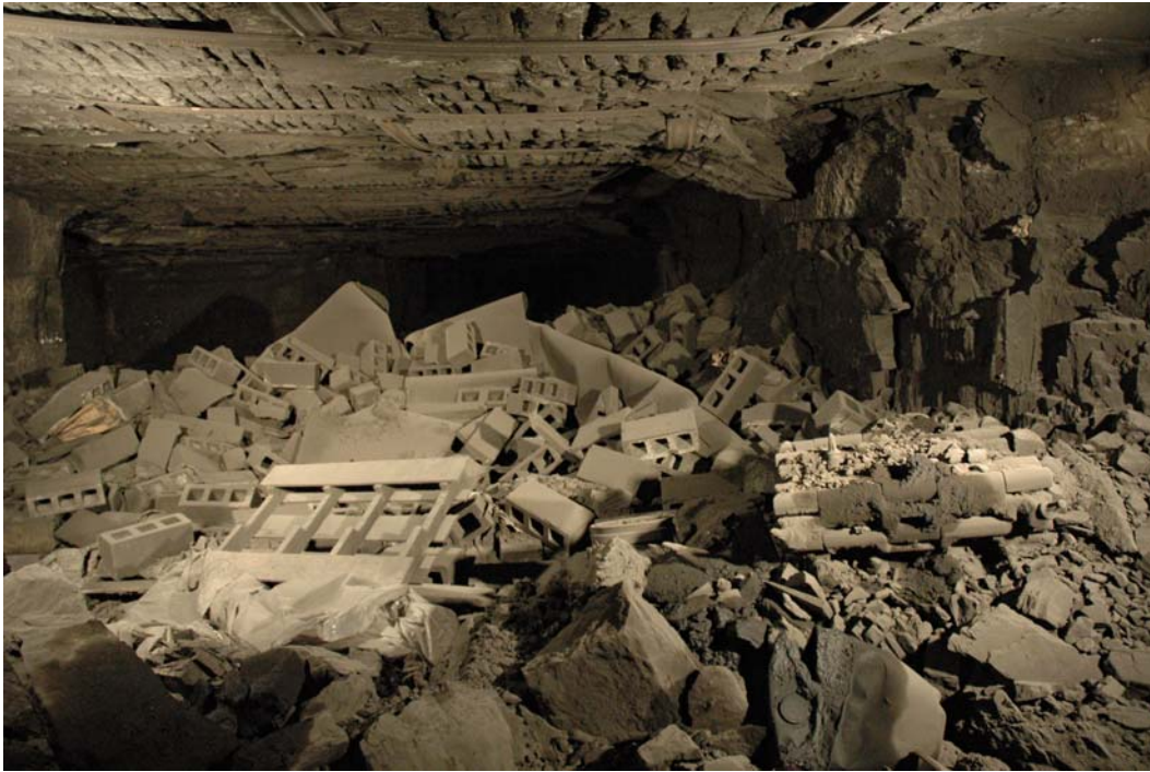
Photograph 11 - Debris from stopping near B Left Section
