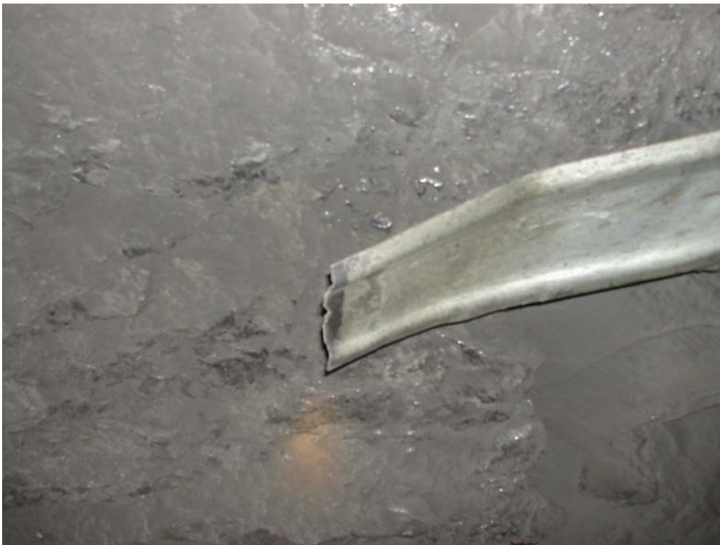
Photograph 6 - Inby segment of roof strap at A Left No. 3 Seal
