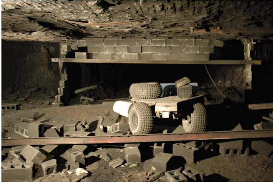
Figure 3 - Personnel Carrier Lodged on Overcast Debris
