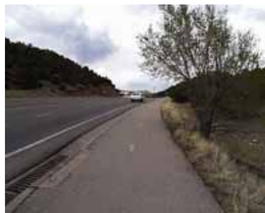
NM 14 Paved Recreational Trail on East Side of Road
