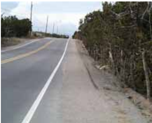
New Paved Shoulders on Mountain Valley Road
