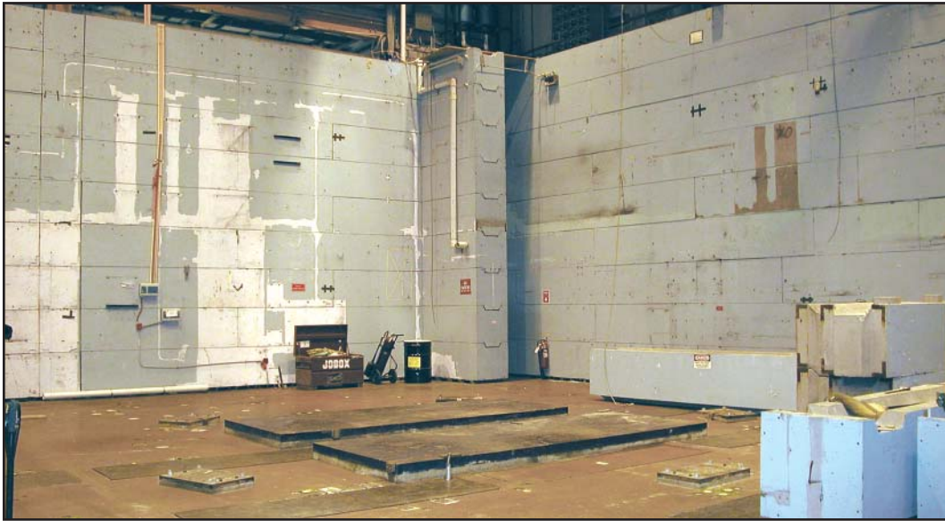
Figure 15. The PBX-M test cell following the completion of its removal.
