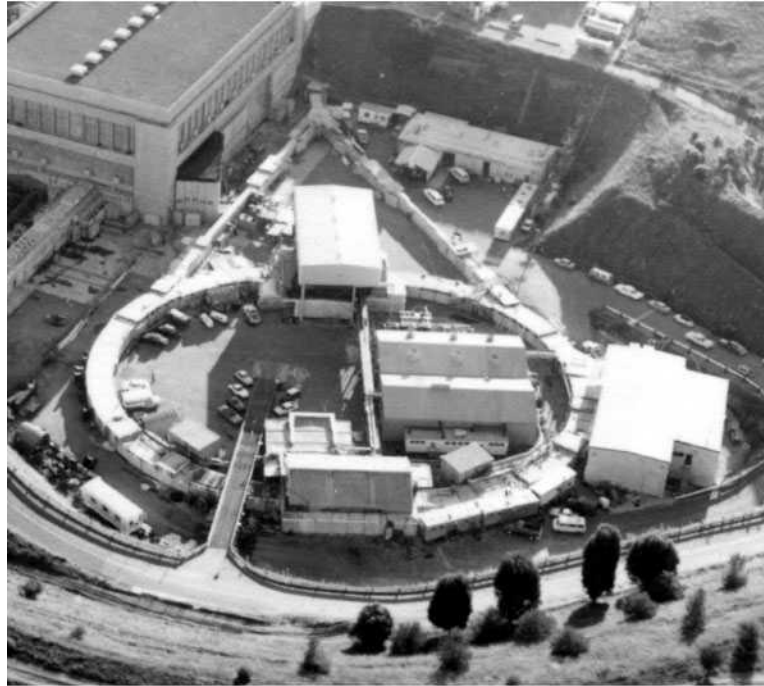
Fig. 2 The SPEAR electron-positron collider at the Stanford Linear Accelerator Center in the early 1970s. The circular building with a diameter of about 80 meters contains the collider itself. The building astride the far end of the ring with the white roof contains the SLAC-LBL detector. Adjacent building contains the control rooms and power supplies for the collider and the detector. Colliders are usually built underground but SPEAR was built above ground because of budget restrictions.
