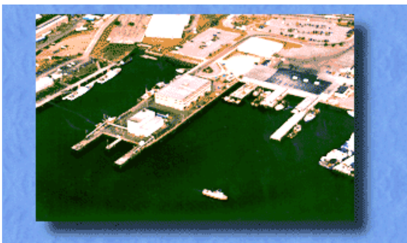
Photo 14. Portland's mixed-use waterfront zoning preserves historical uses such as fishing and boatbuilding in proximity to tour boats, residences and office buildings.
