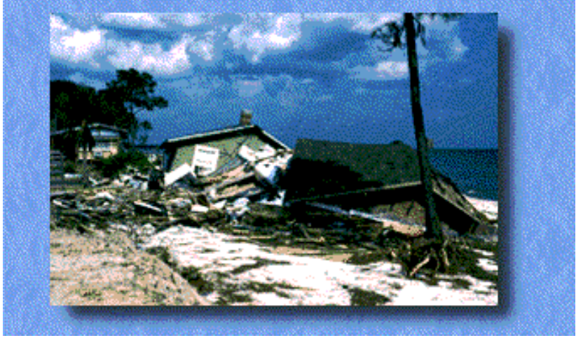
Photo 3. Hazard avoidance and reduction are increasingly emphasized as disaster-related costs rise.
