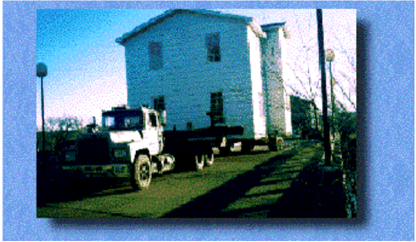
Photo 11. The truck is towing a home to an area of lower risk for erosion. Relocation of structures is a preventive mitigation strategy.
