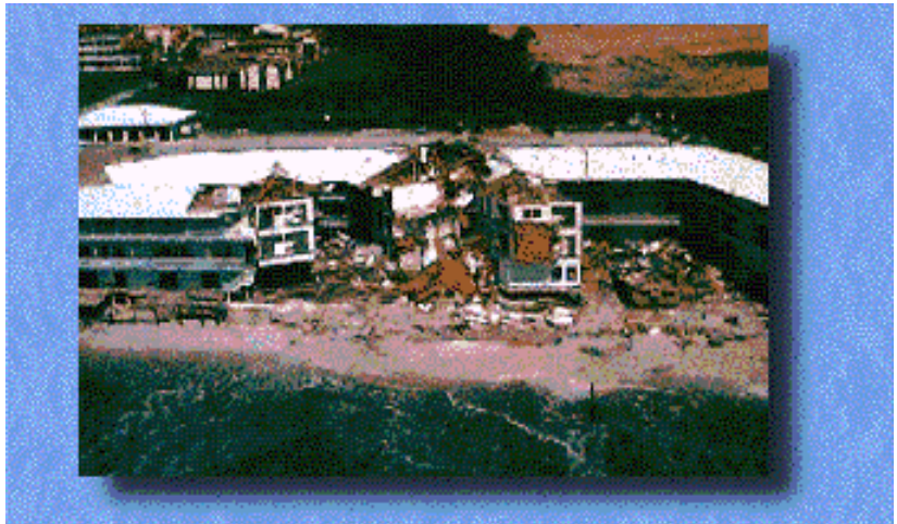
Photo 9. This condominium complex built on the shoreline displays damage caused by the high winds of a hurricane.
