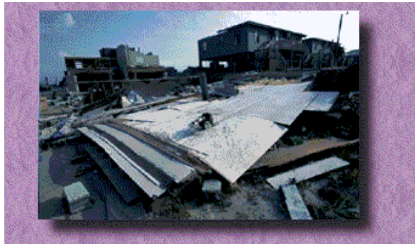
Photo 1. A hurricane damaged these North Carolina coastal homes.
