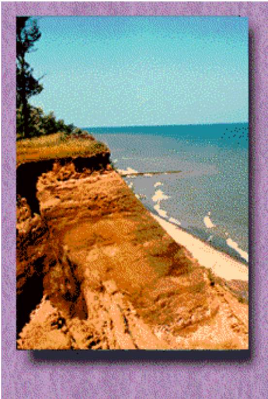
Photo 6. Erosion occurs not only on sandy
