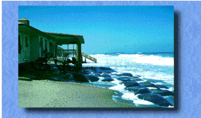
Photo 17. To prevent coastal structures from wave action, as shown above, North Carolina requires coastal structures to be set back from the shoreline at a distance related to long-term erosion rates.
