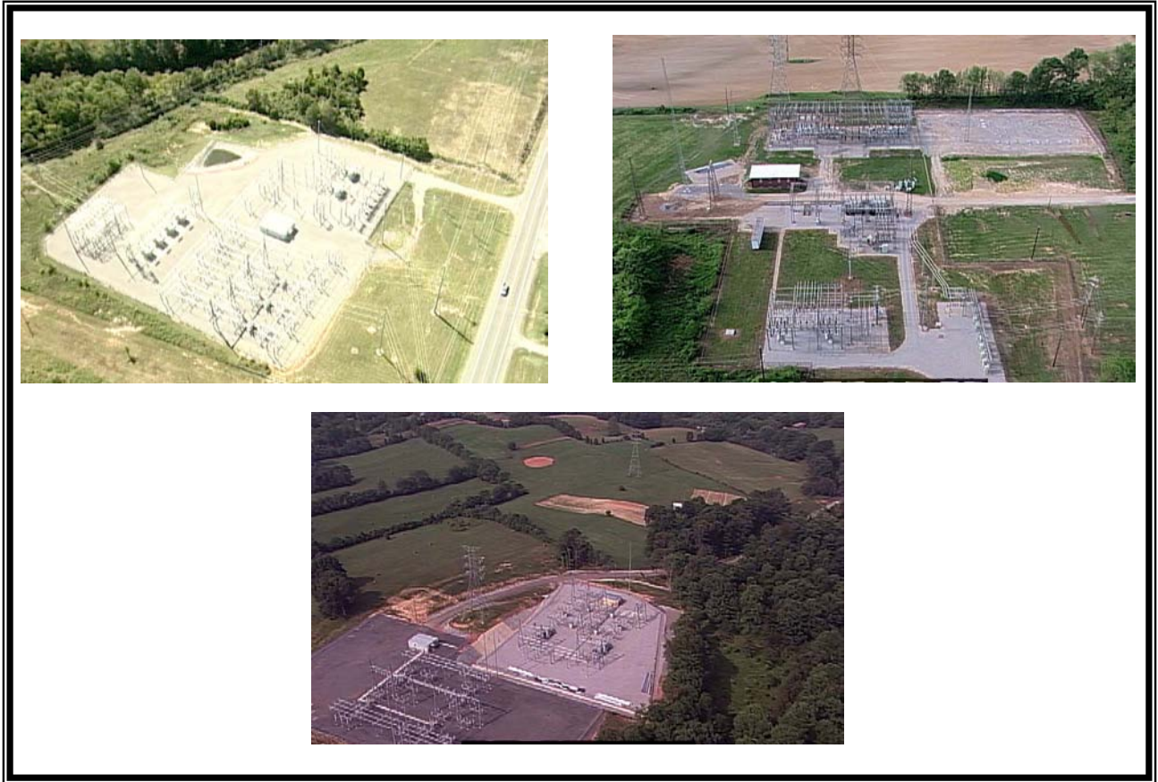
Figure 2-11. The Design of Other Existing TVA Switching Stations
