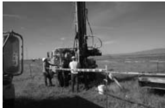
A well decommissioning crew and rig are set up in central Hanford.
