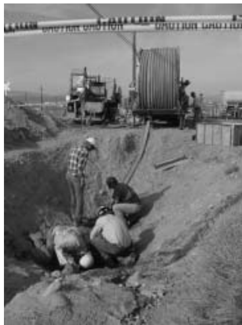
Hanford's groundwater remediation involves a variety of activities including mortar-lining of leaky water pipes.
