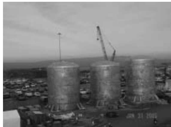
Waste Treatment Plant construction — Pre-treatment Facility vessels.
