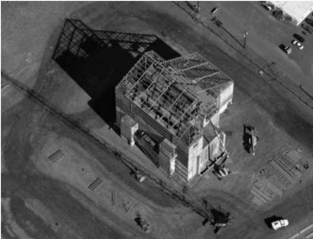
Aerial view of roof construction of the H Reactor.
