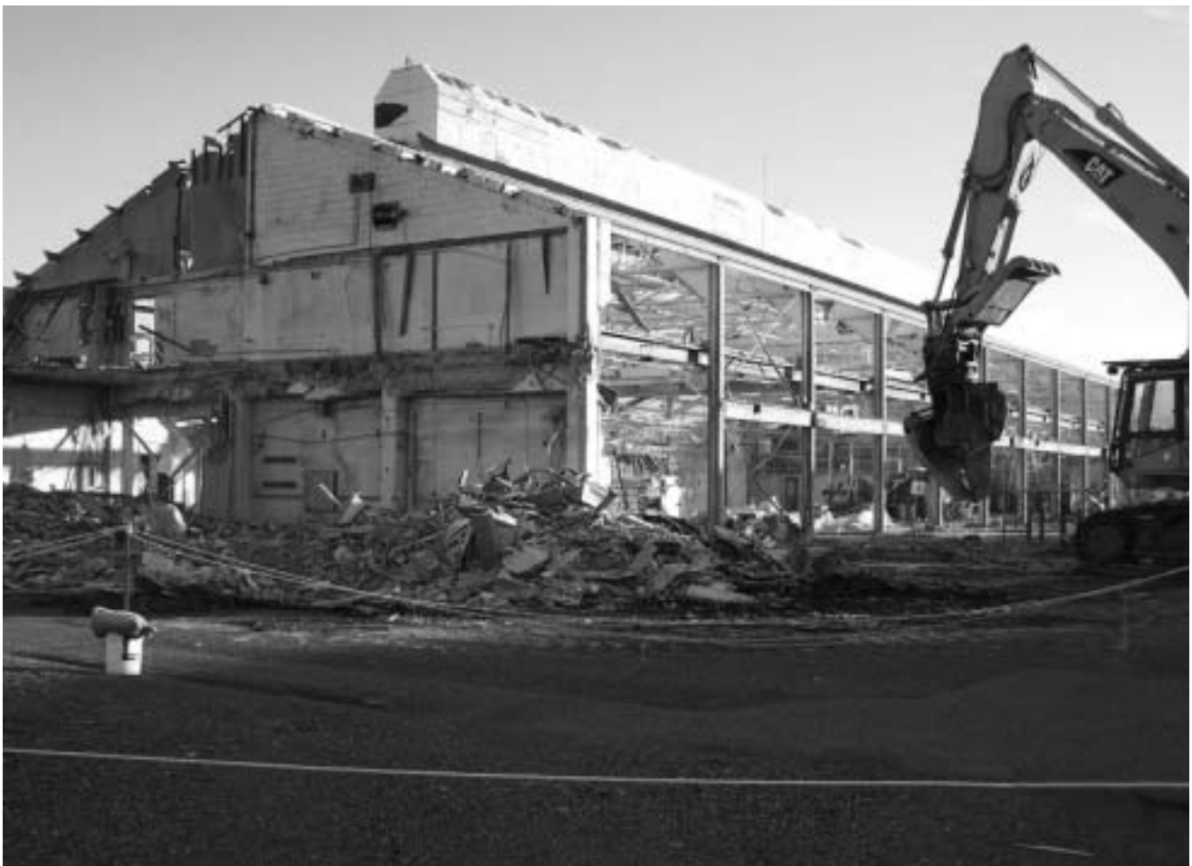
Demolition of 314 Building.
