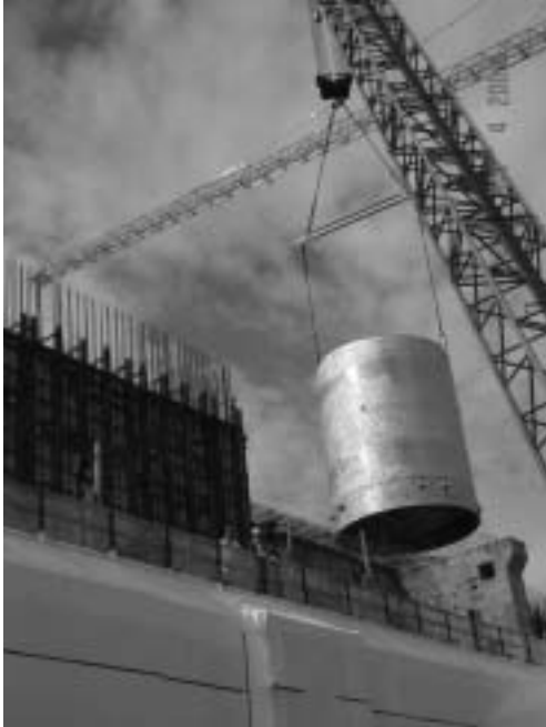
Waste Treatment Plant construction vessel installation.
