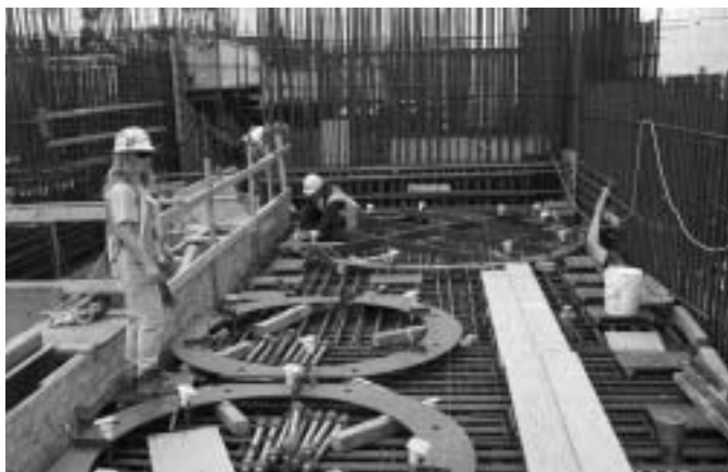
Waste Treatment Plant construction.
