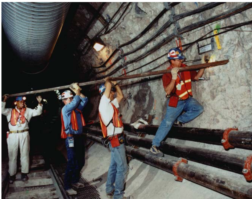
Heater element installation for thermal testing in the cross drift, April 2001
