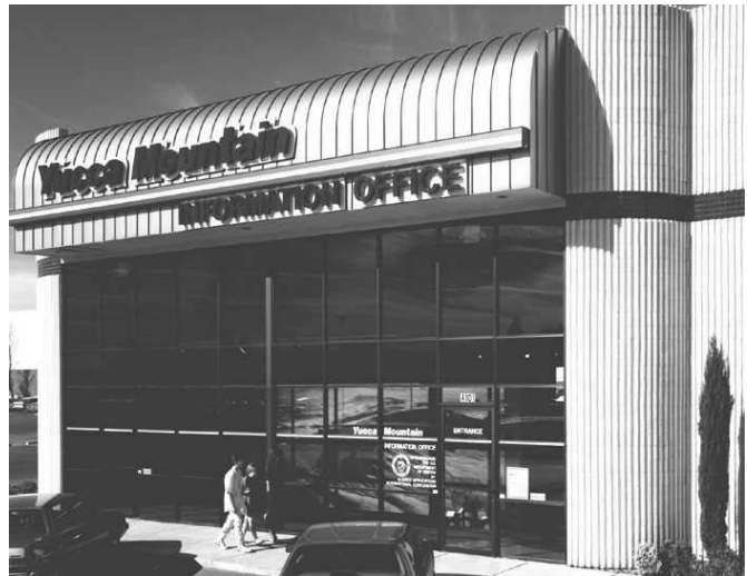
Exterior view of the Yucca Mountain Science Center and Information Office, Las Vegas, NV
