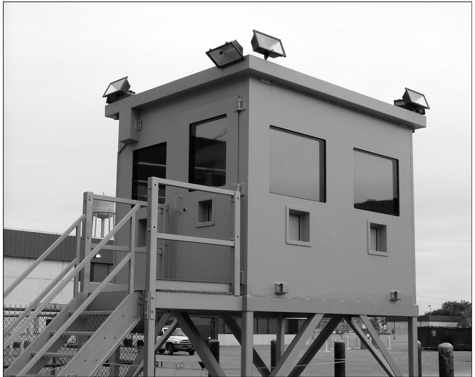
Figure 1: Example of a Bullet-Resistant Structure
