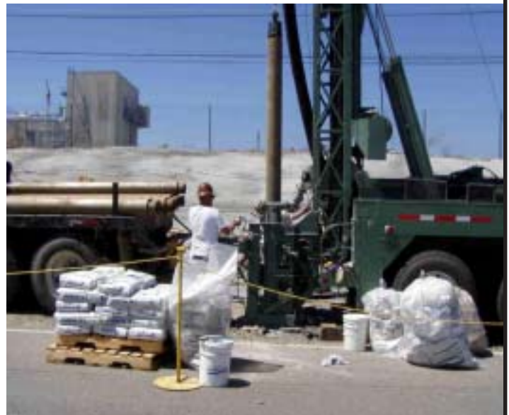
Hanford monitoring well construction.
