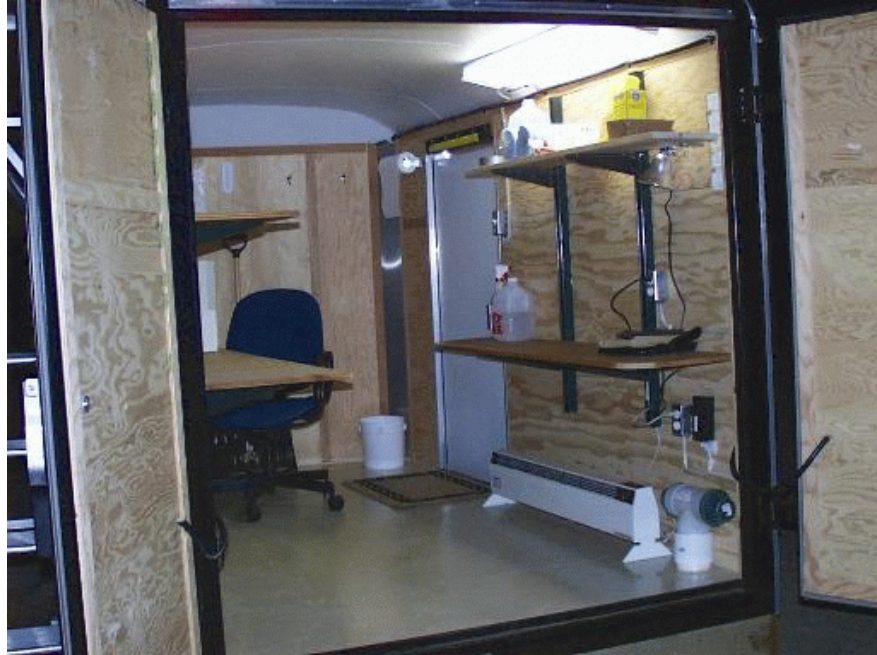
Figure 6. The finished interior. Fresh air inlet located bottom right.
