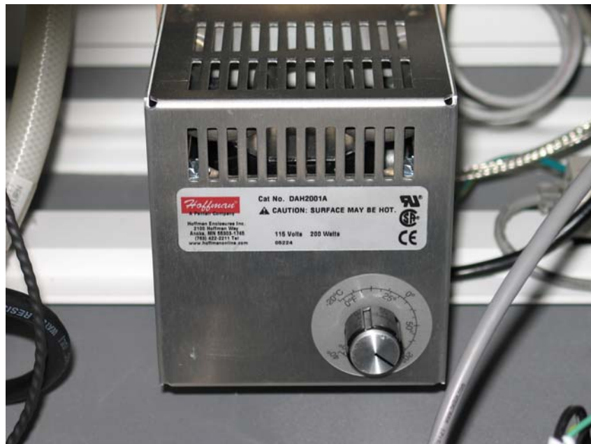
Figure 16. Environmental Enclosure heater.
