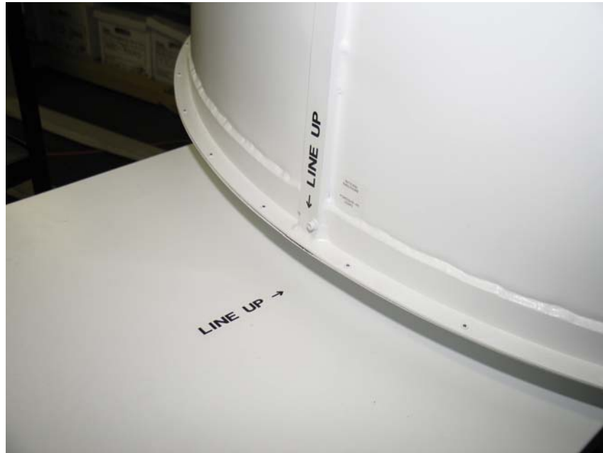
Figure 26. Proper rotational alignment of the antenna.
