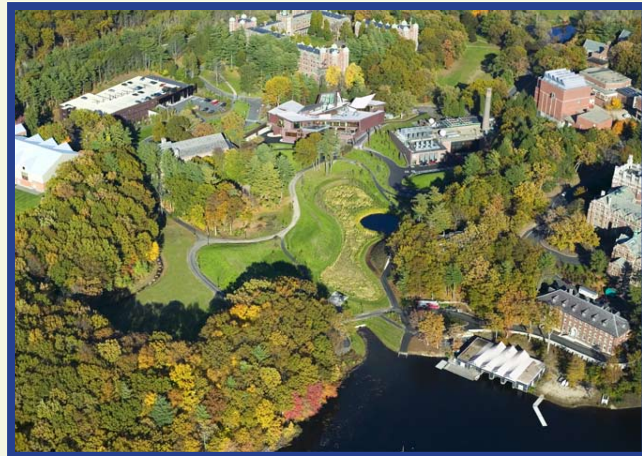
BROWNFIELD TO GREENFIELD, WELLESLEY, MASSACHUSETTS. MICHAEL VAN VALKENBURGH ASSOCIATES, INC., CAMBRIDGE, MASSACHUSETTS AND NEW YORK, NEW YORK.
