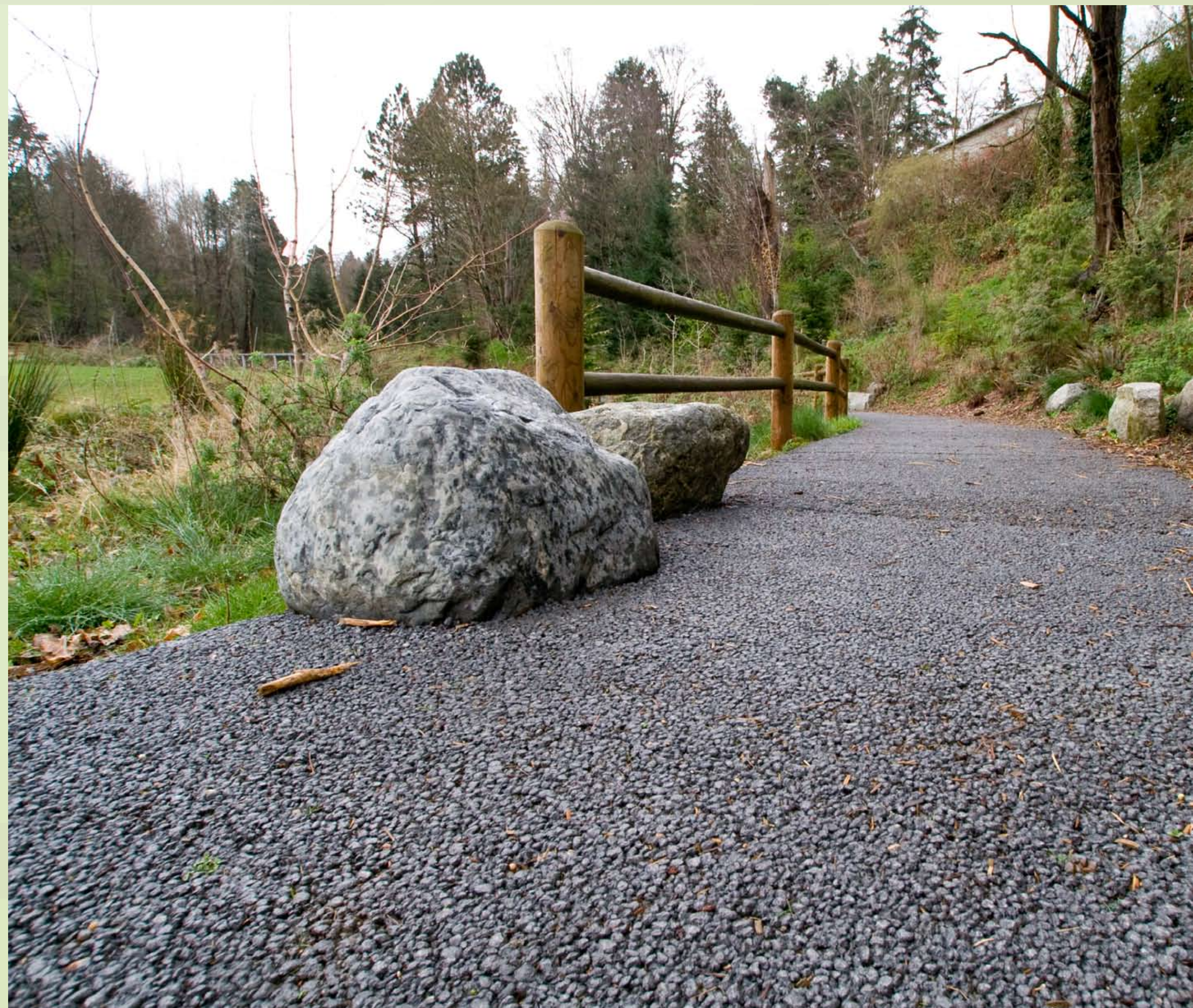
Ravenna Park, Seattle: Permeable paving was used for footpaths at the entrance of the popular nature walk along the ravine and it's recently daylighted creek.
