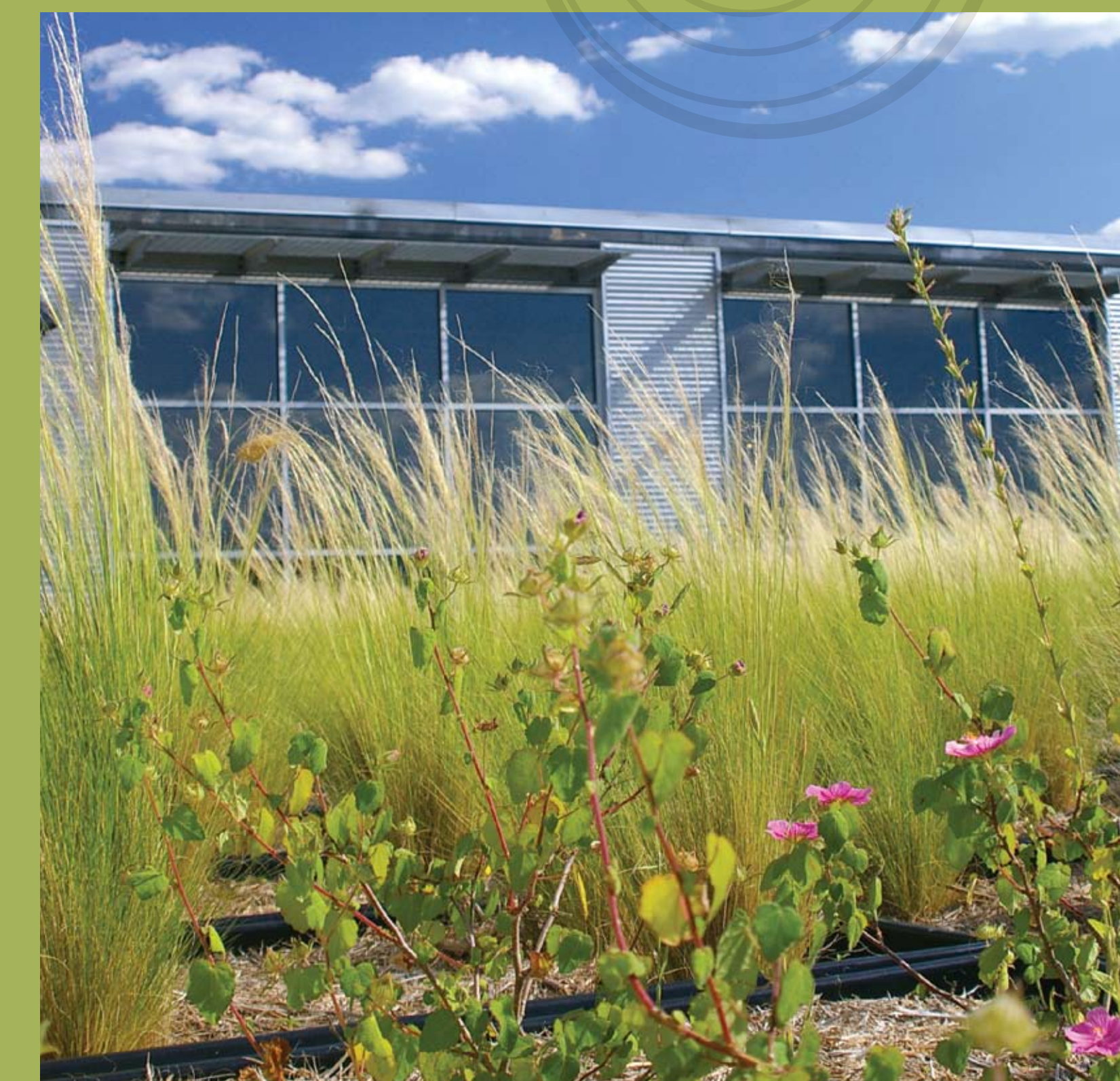
This Austin, Texas, green roof helps cool the building below and controls storm water runoff. Wildflower Center photo by Philip Hawkins
