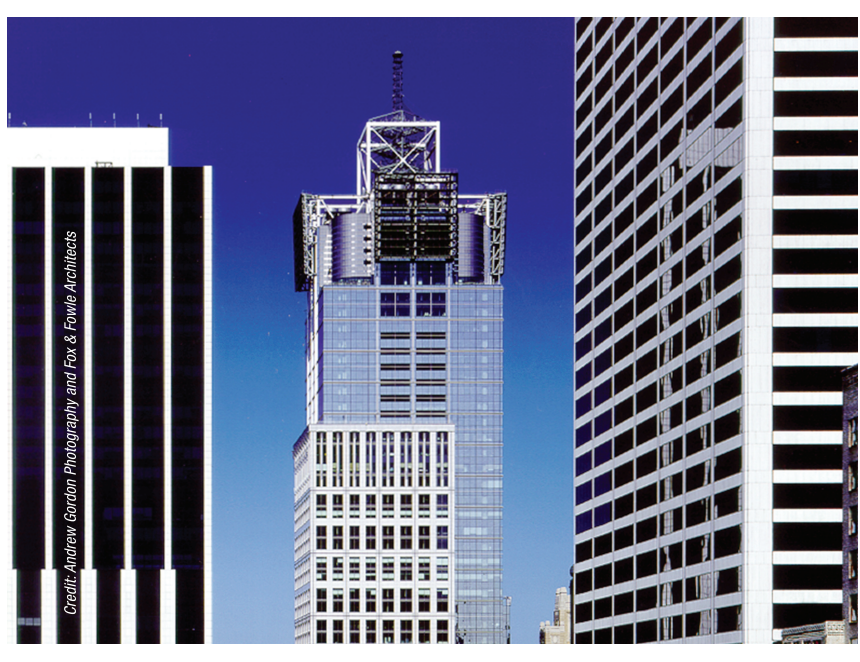
▲ The 4 Times Square building in NEW YORK CITY has a photovoltaic "skin" on the upper floors, in which thin-film PV panels replace traditional glass cladding material. The system provides enough energy to power the equivalent of five to seven homes.
