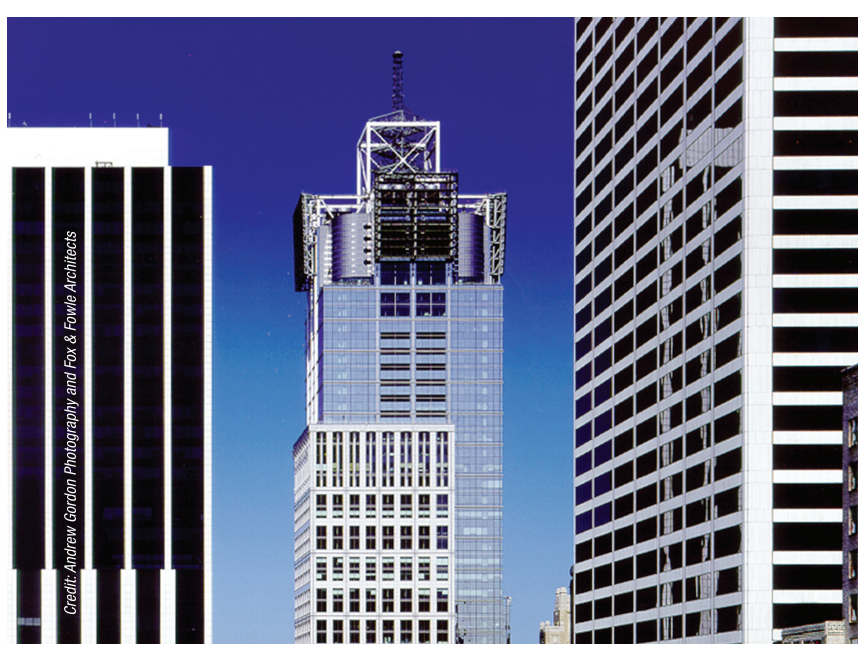
▲ The 4 Times Square building in NEW YORK CITY has a photovoltaic "skin" on the upper floors, in which thin-film PV panels replace traditional glass cladding material. The system provides enough energy to power the equivalent of five to seven homes.
