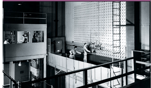
Operators working in the ORNL Graphite Reactor
