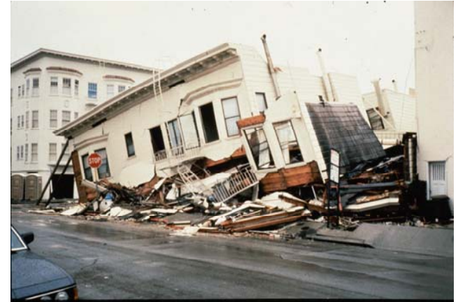
1994 Northridge Earthquake, Los Angeles (NIST)
