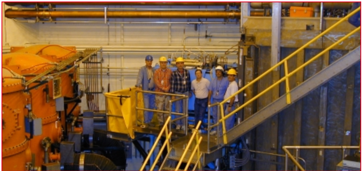
Staff responsible for the installation of the third and final long-pulse ion source on the NSTX neutral beam. From left: Paul Ernst, Len Halvorsen, Martin Wisowaty, Mark Cropper, Kris Gilton, and Ed Bush.
