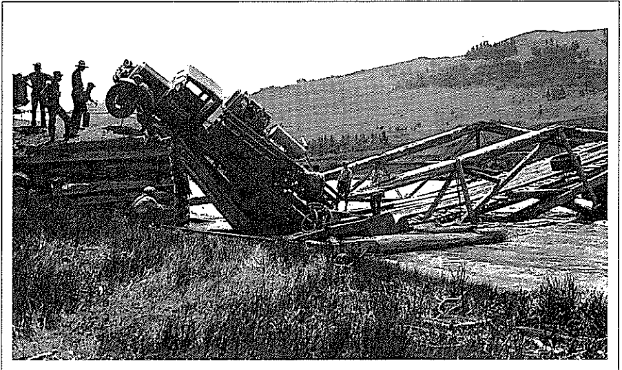
Above: The Lamar River Bridge broken by overload, 1932. Below: Gardner River Bridge, 1917.
