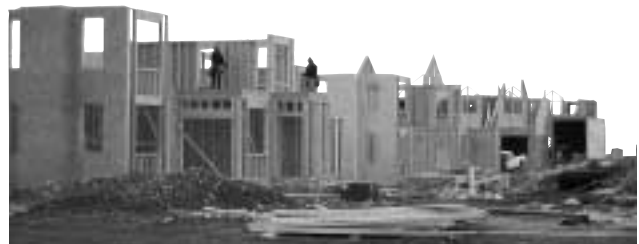
Condominium construction near Grand Targhee, Idaho. Photo courtesy Greater Yellowstone Coalition.
