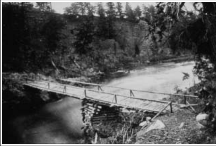
Baronett Bridge across the Yellowstone River. Photo by William H. Jackson, 1871. NPS photo archives.
