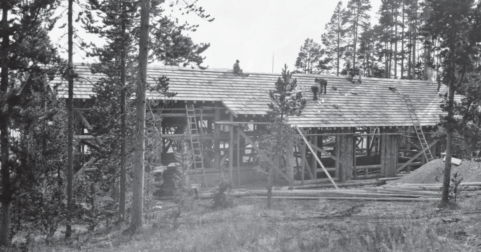
Construction of the Lake fish hatchery building in 1928.
